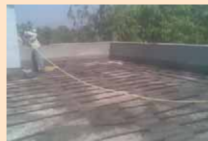
Laying out the coil of pipes above RCC slab with screed below tiling at the time of construction of terrace
