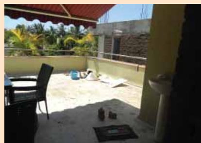
Completed terrace with water pipes below tiling and high albedo paint above
