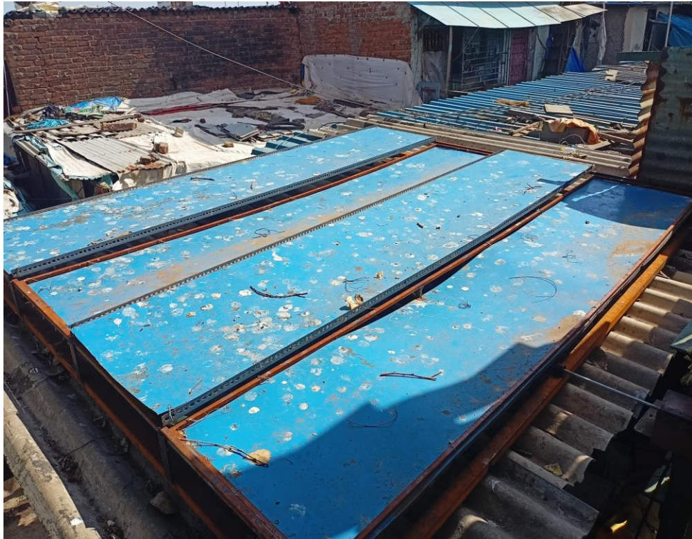
Alufoil Sliding (on a tin-roofed house)
