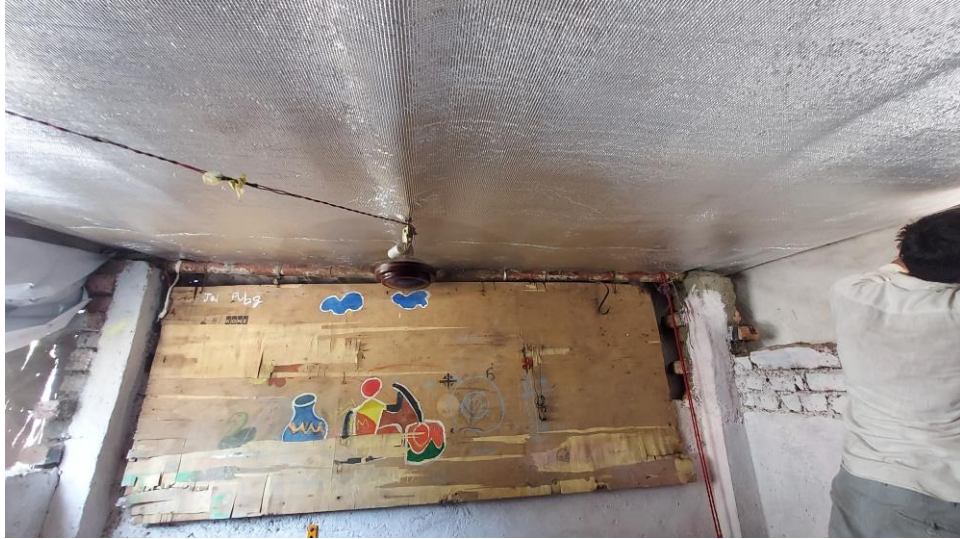
Alufoil Static (under a tin-roof)
