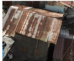
Corrugated Tin roof
