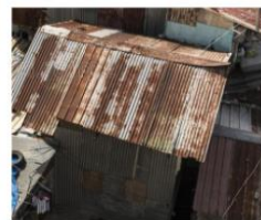
Corrugated Tin roof
