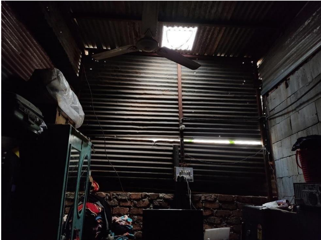
Dormer Window: Indoor view
