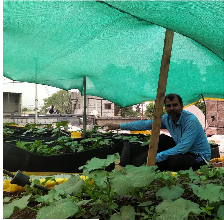
Rooftop Garden Installation
