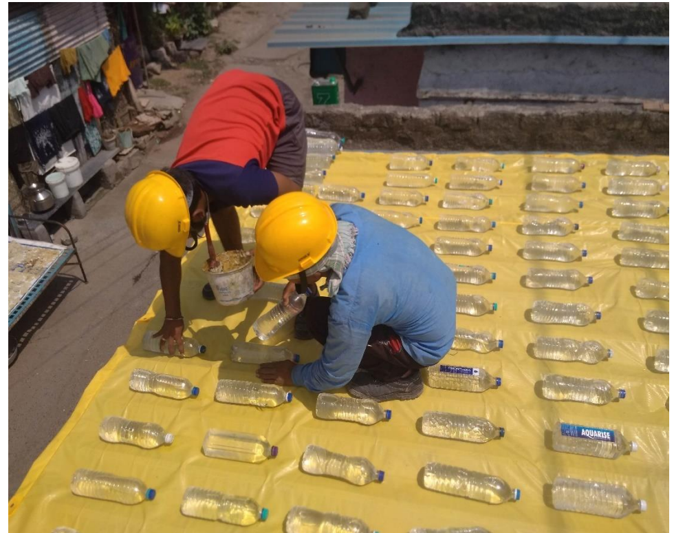
Water filled PET bottle- Installation
