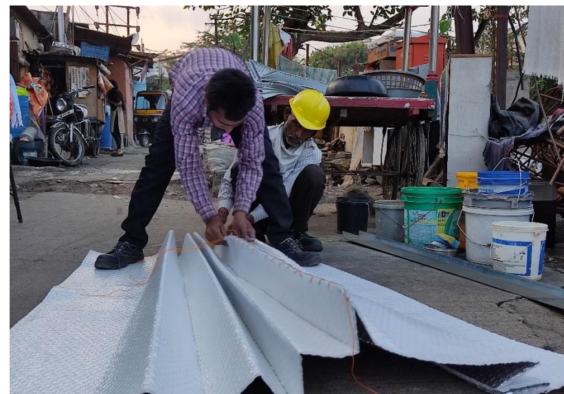
Onsite fabrication of Alufoil Installation
