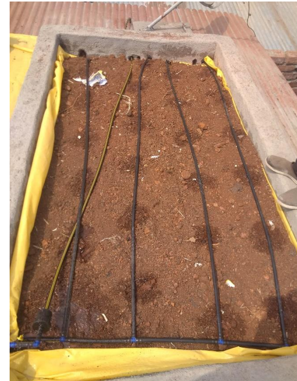
Rooftop Garden: Irrigation System
