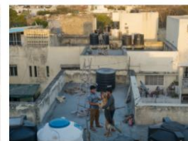
Concrete slab roof
