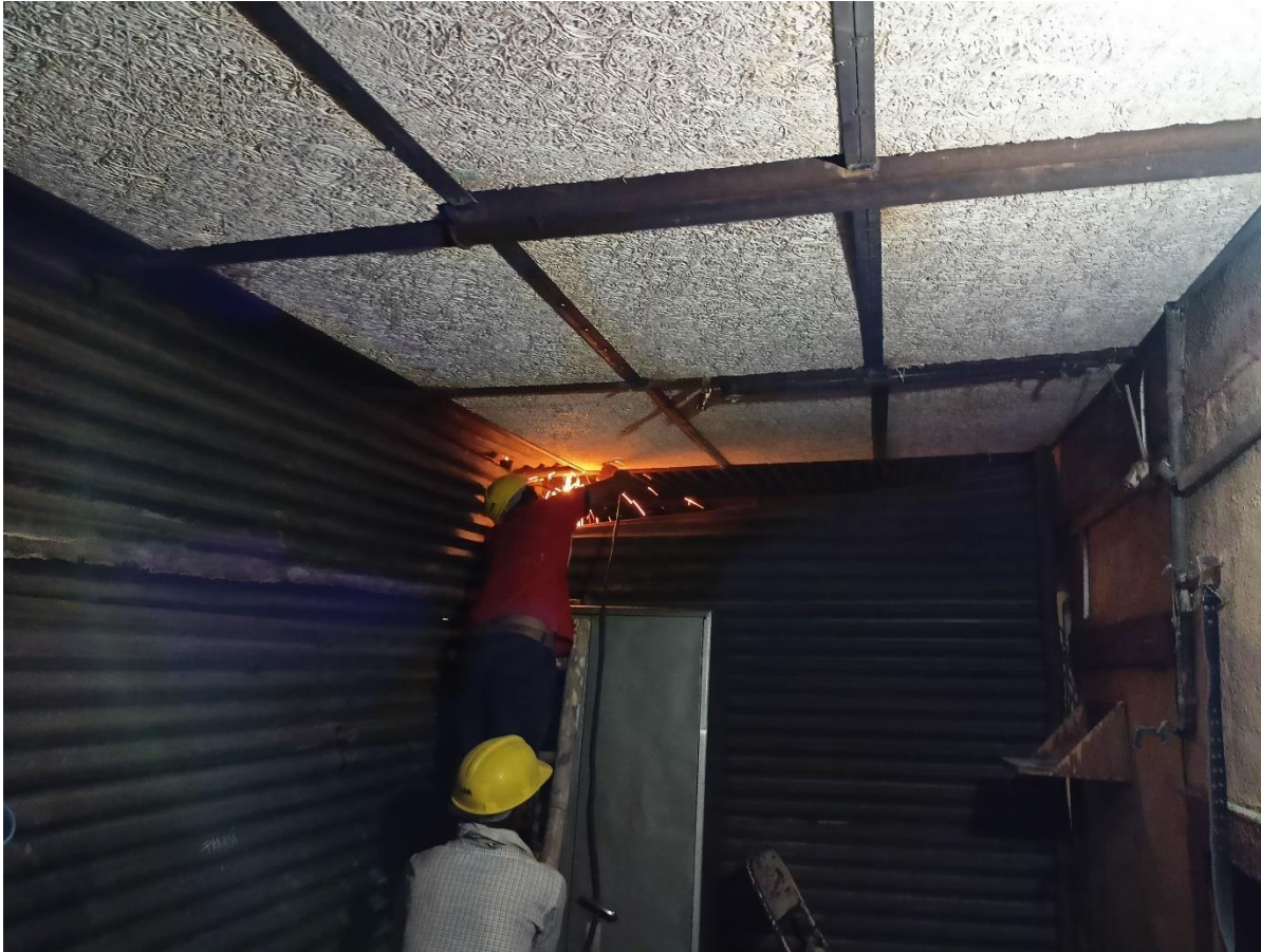
Wood Wool Panel Installation
