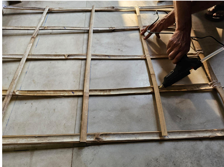
Fig 24: Making Bamboo Frame
