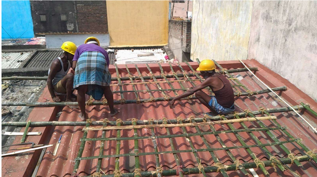
Fig 37.4.2-11 : Bamboo trellis making process
