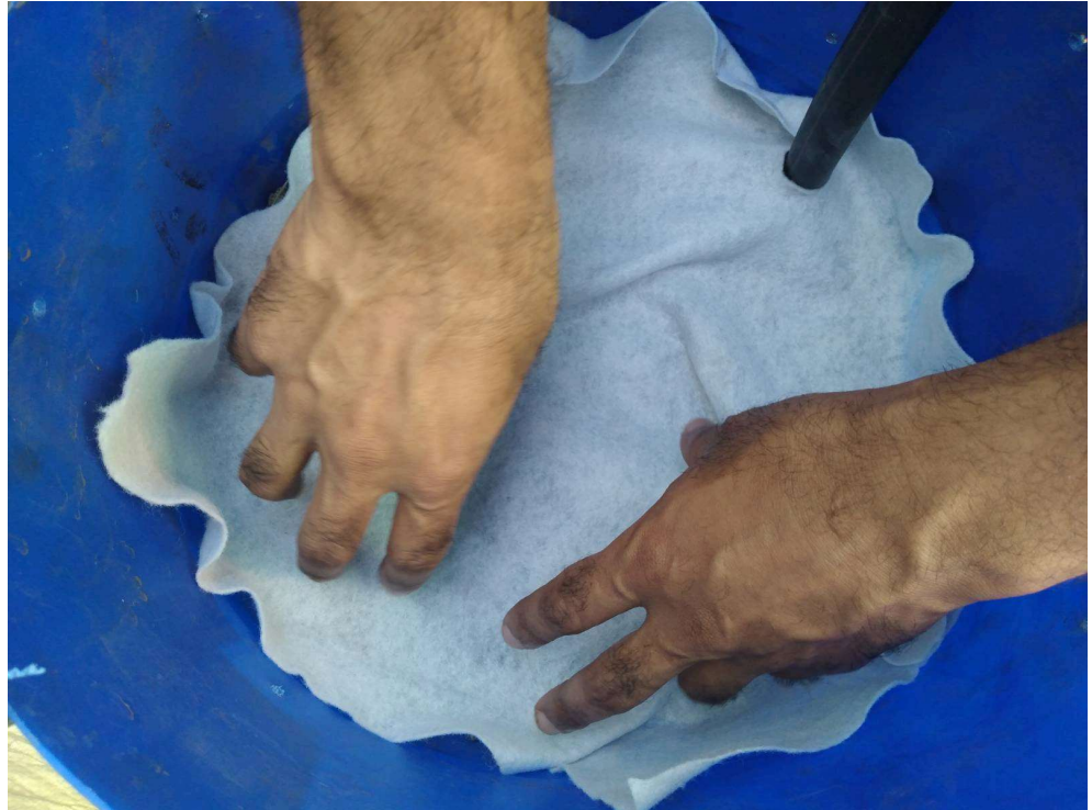
Fig 37.4.2-9 : Place Geofibre on top of concrete chips
