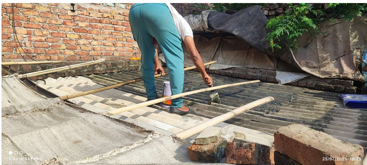
Fig 37.6.3-1 : Applying Of Adhesive Above The Roof
