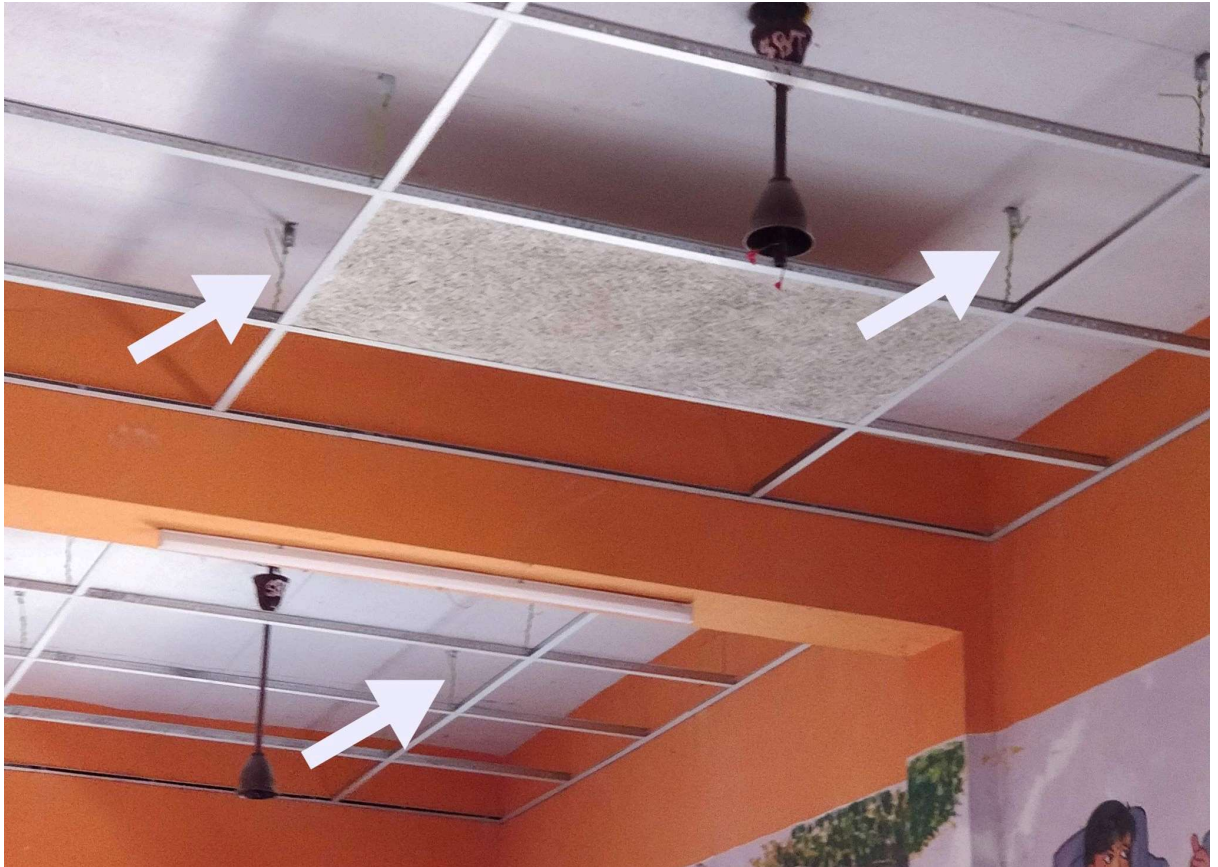
Fig 37.3.2-3 : Extra roof support
