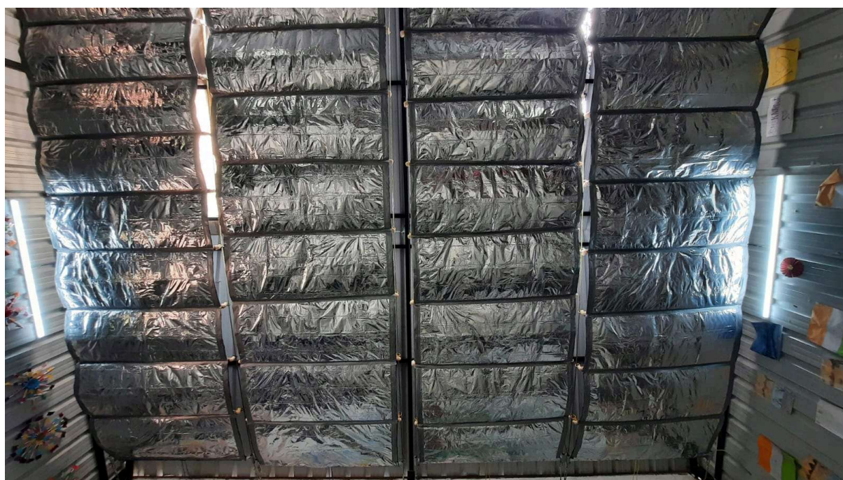
Fig 37.1.3-8 : Fractals (in open position) covering the underside of the Roof.
