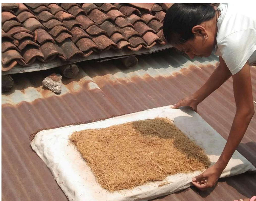
Fig 37.2.2-12: Sun-dry the panels
