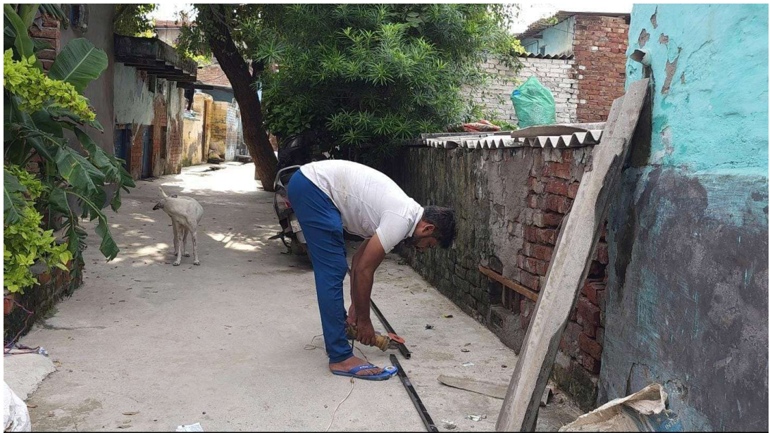
Fig 37.5.2-2 : Cutting Of MS Strip
