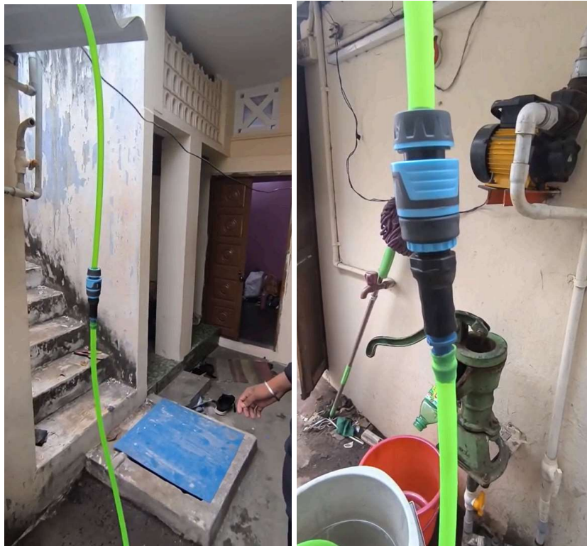
Fig 35.3.4-3 : Easy Removable Hose Pipe Connector
