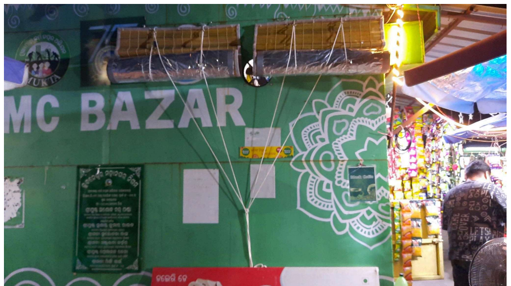
Fig 22.1.3.6-1 : Vertical Cane Blind Installation
