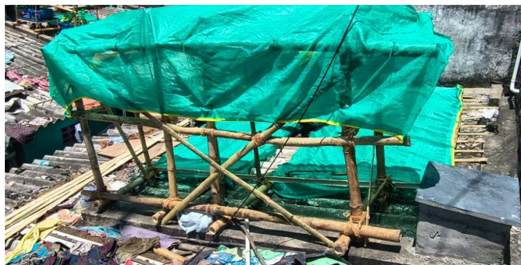
Fig 37.4.2-15 : Scaffolding after finishing all works
