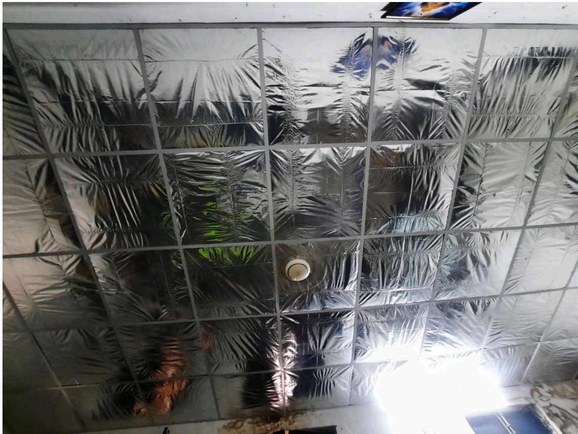
Fig 22.1.6-1 : MLP Static Panel Installation at Office Space
