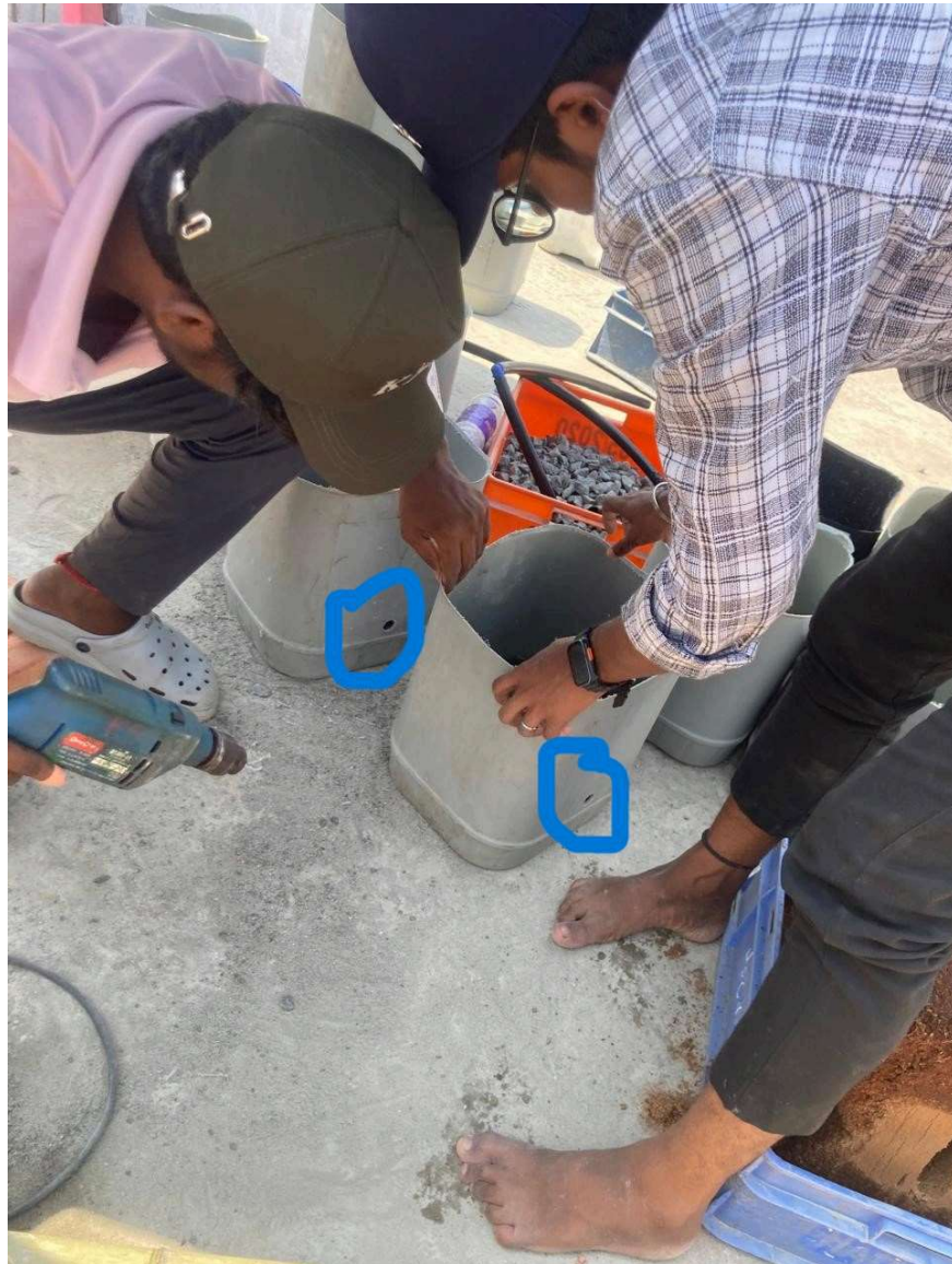
Fig 37.4.2-3 : Making 20mm hole with driller
