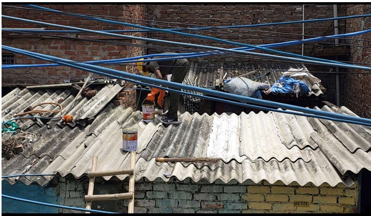
Fig 37.5.3-1 : Applying Of Adhesive Over The Roof
