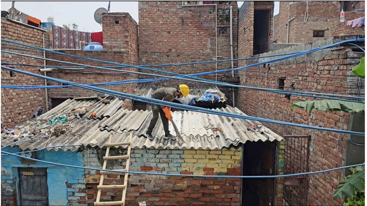
Fig 37.5.1-1 : Cleaning Of Roof
