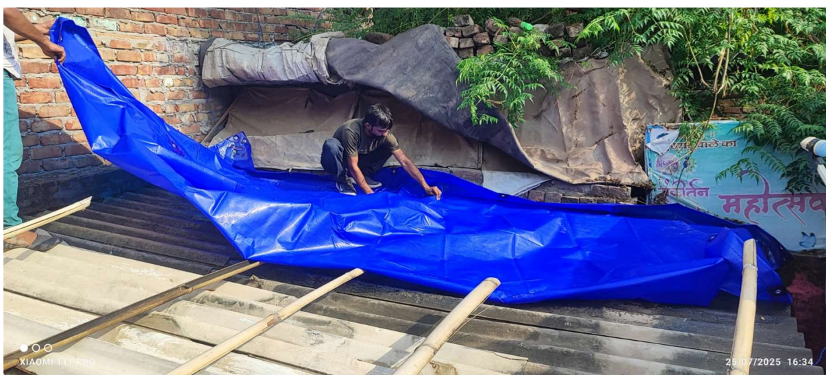
Fig 37.6.3-2 : Placing Of Silpaulin Above Roof
