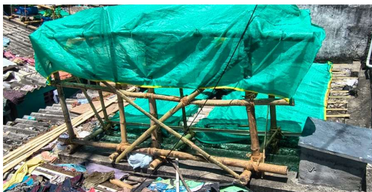
Fig 35.3.3-2 : Scaffolding Structure with Shade Net
