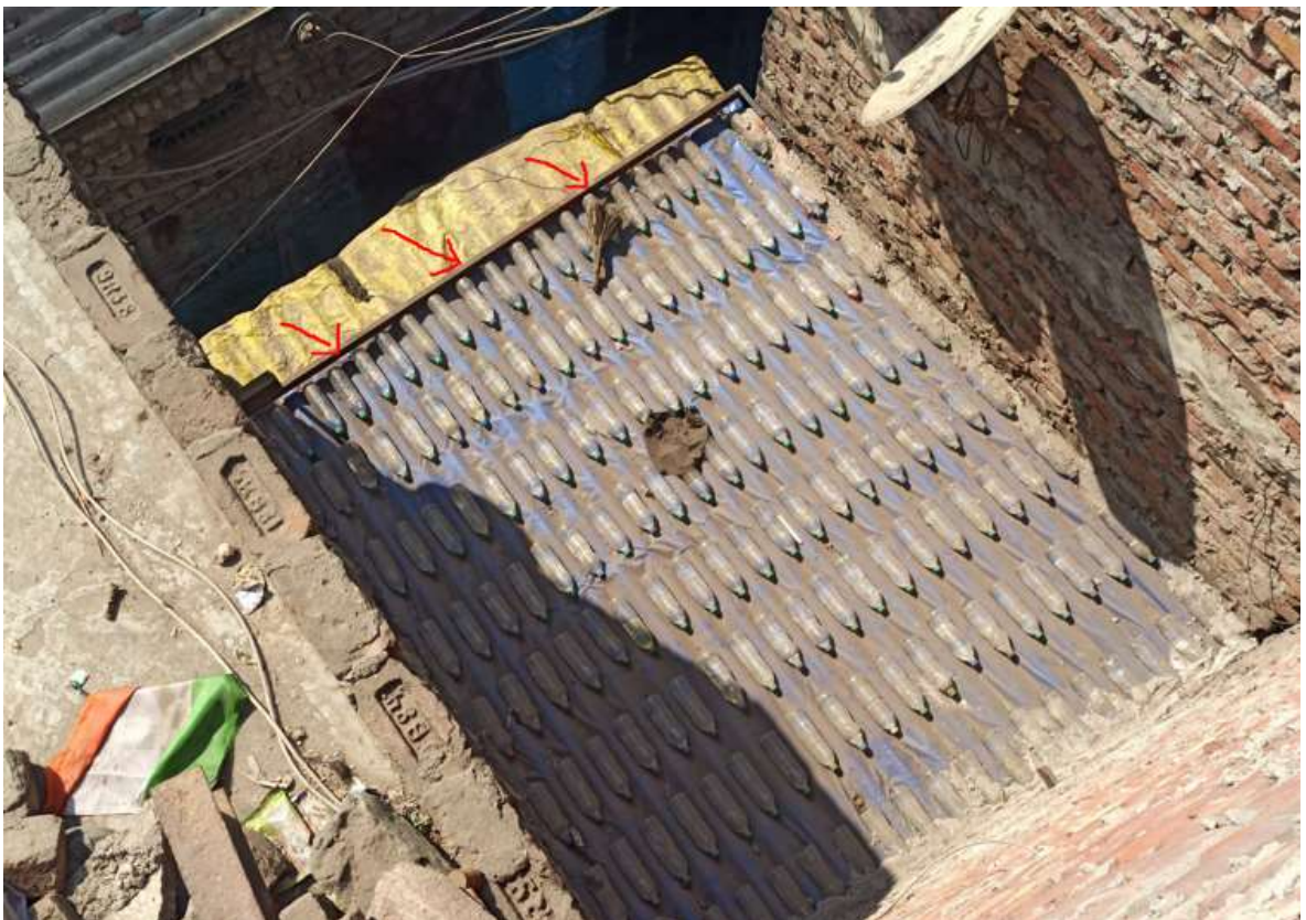
Fig 37.5.3-9 : Top View After MS Strip (highlighted by red arrows) Installation
