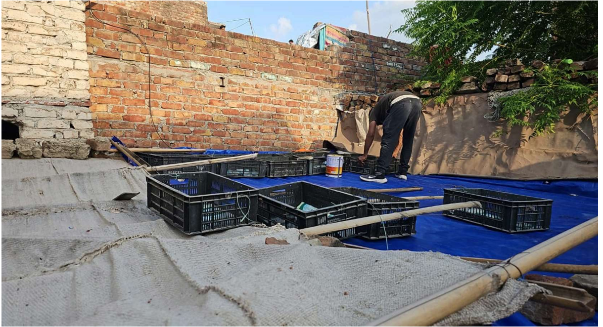
Fig 37.6.3-3 : Placing Of Crates Above Roof
