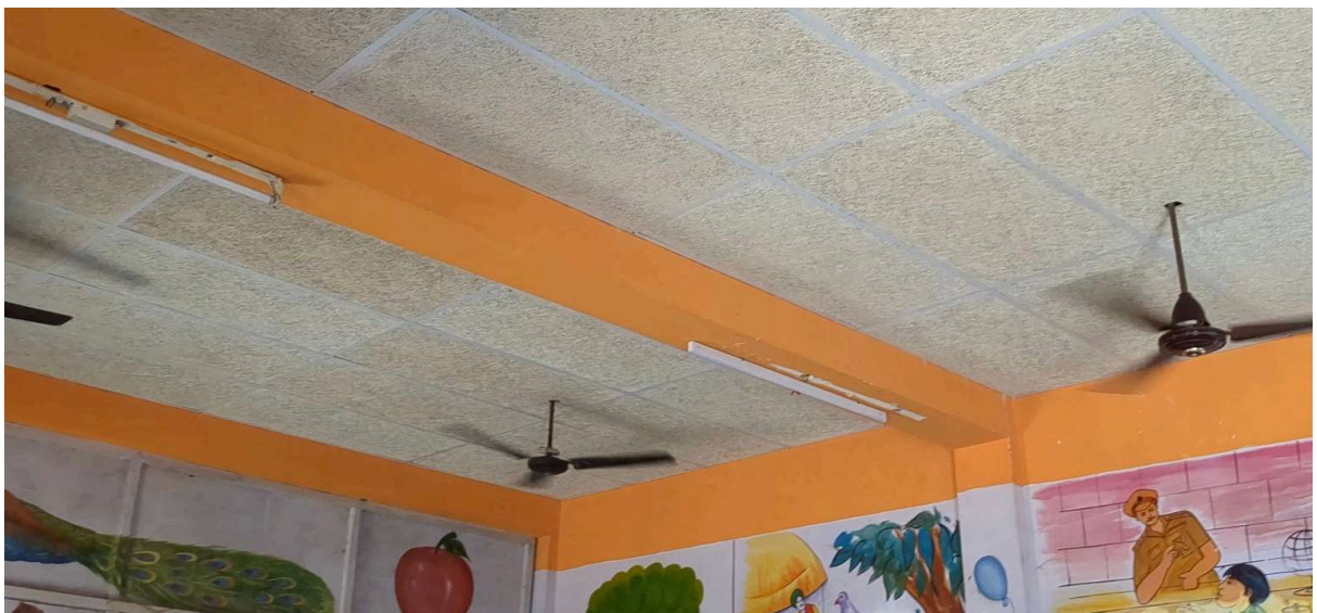
Fig 37.3.2-6 : Steel alloy support framework with panels in place
