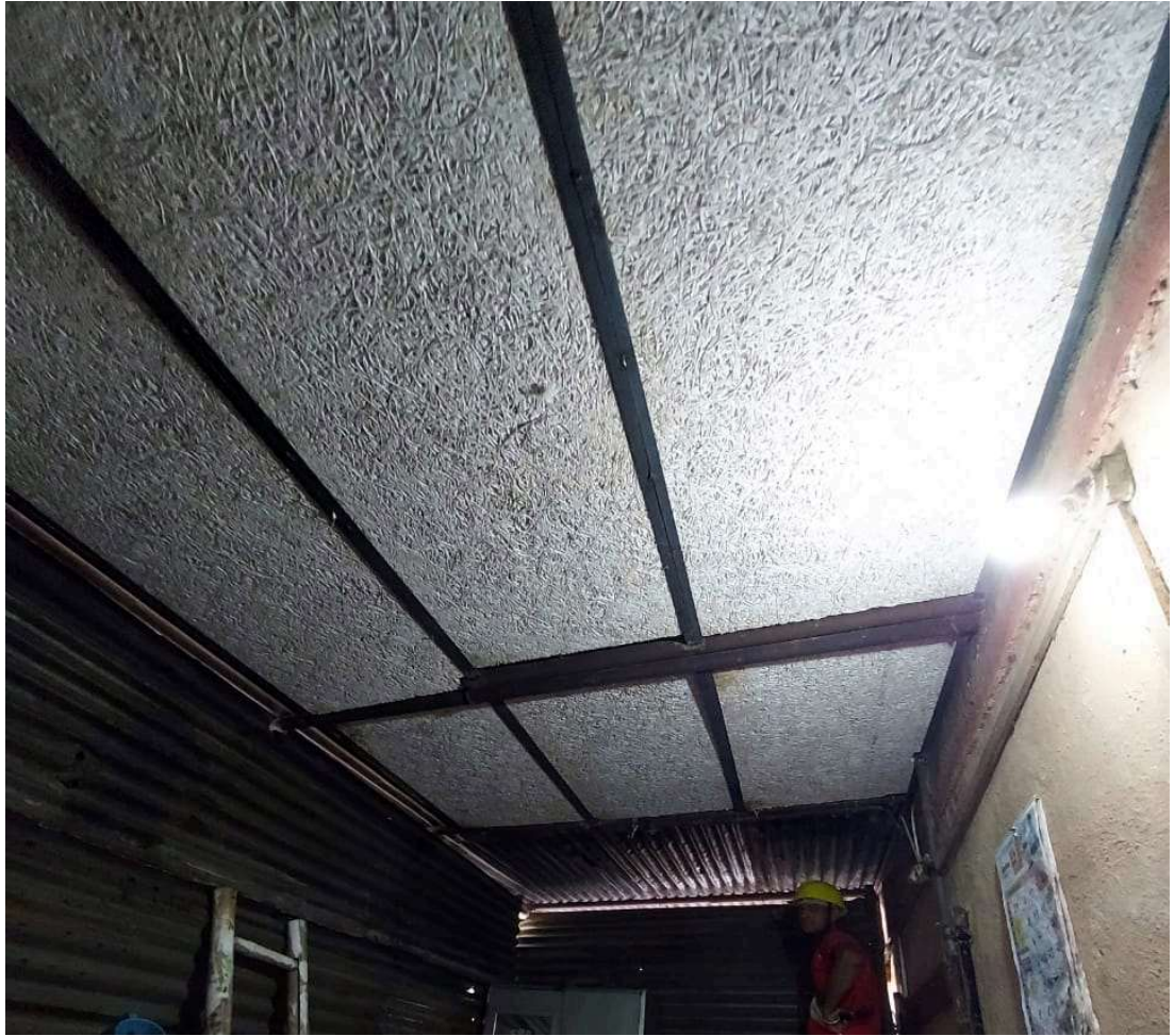
Fig 37.3.2-5 : MS support framework with panels in place
