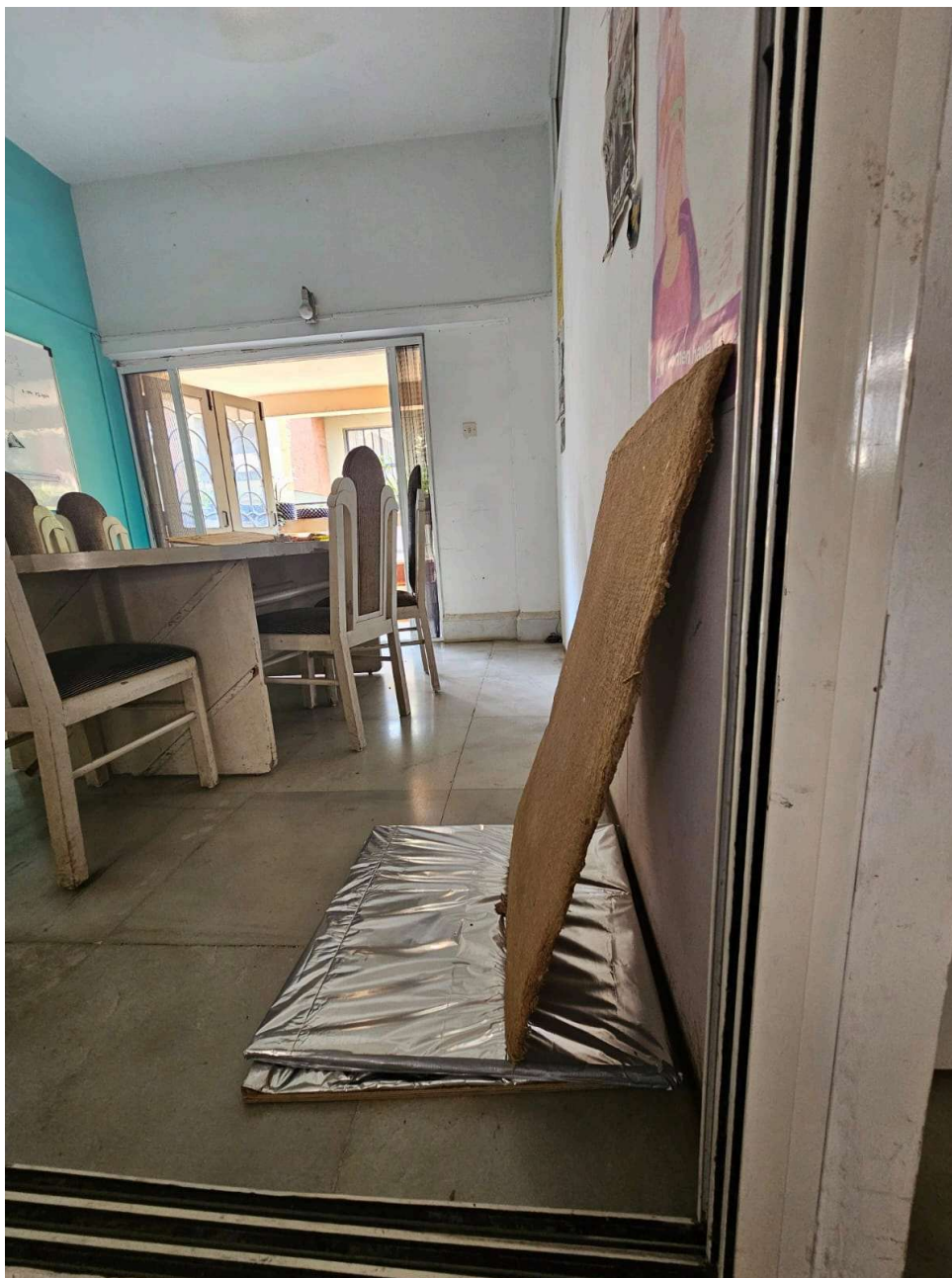
Fig 37.2.3-5 : Ensure panels are stored on raised pallets
