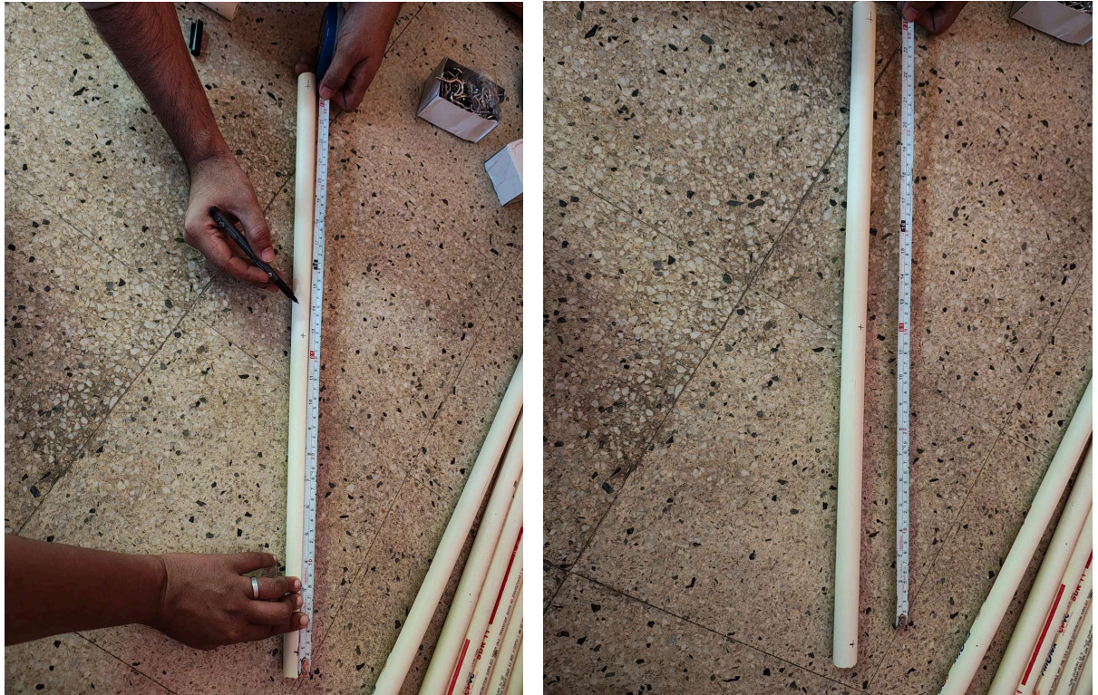
Fig 37.7.2-13 : Marking of points to attach hooks.
