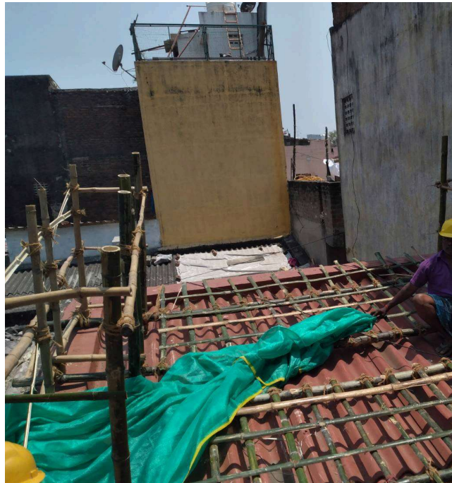
Fig 37.4.2-12 : Green net attaching to the Bamboo trellis
