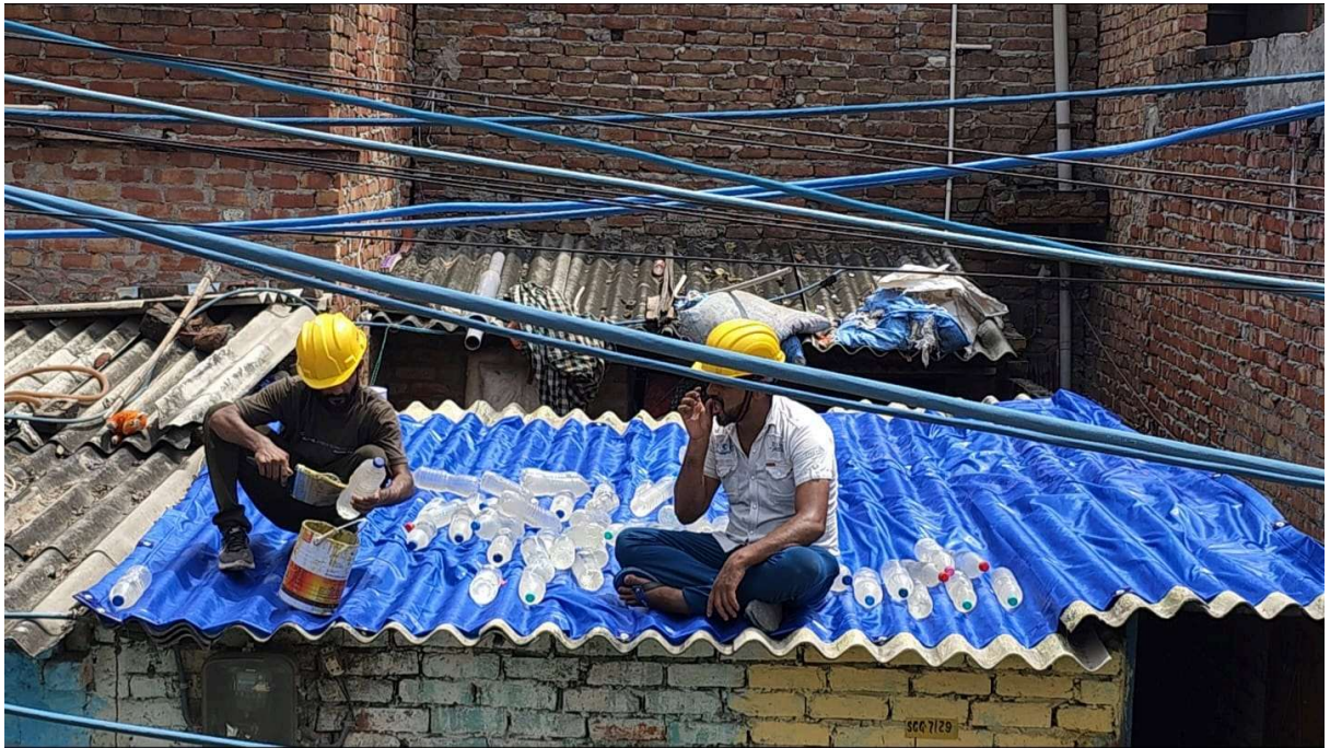
Fig 37.5.3-4 : Application Of Adhesive Along The Bottle Side Which Touches The Roof
