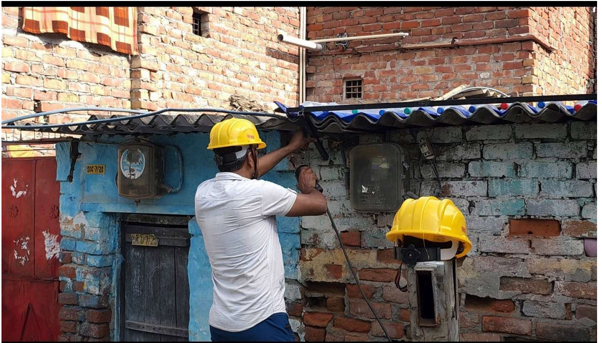
Fig 37.5.3-7 : Securing Of MS Strip Through Welding
