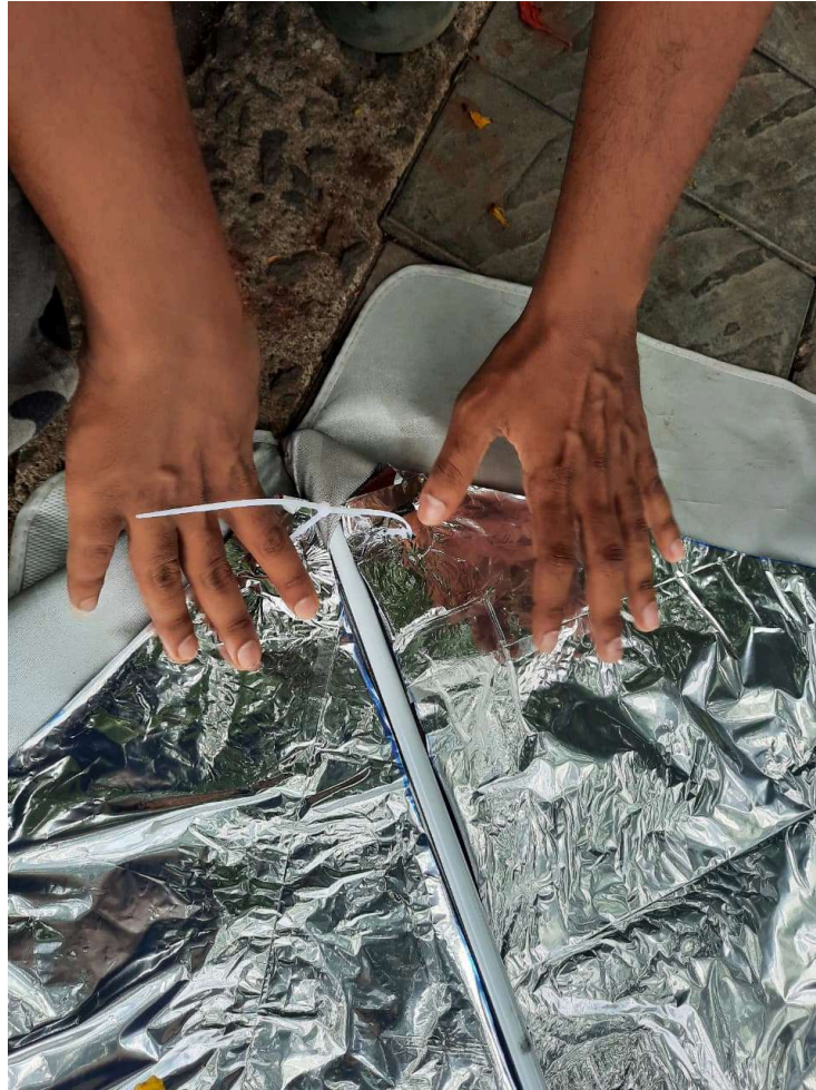
Fig 35.8.1-6 : Securing MLP Panels using Plastic Ties
