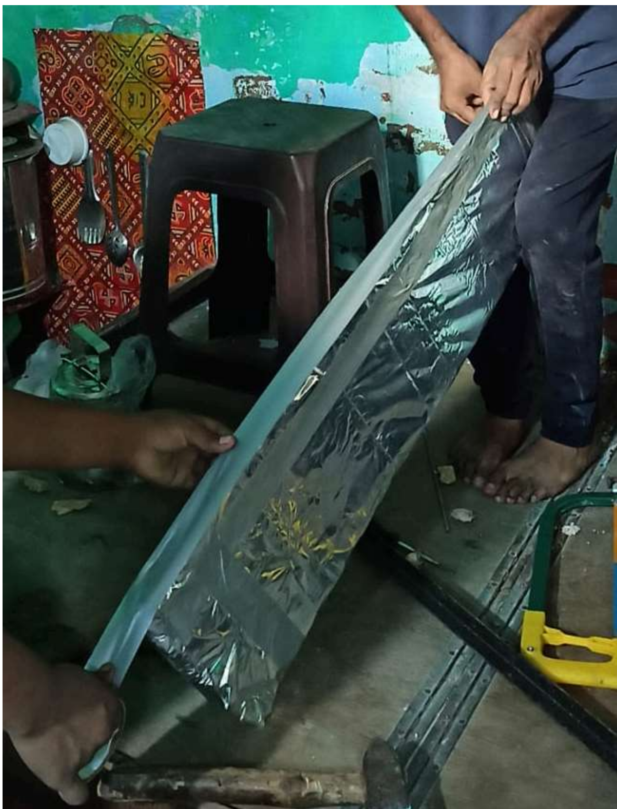
Fig 37.2.5-6 : Tape the cut end with aluminium tape
