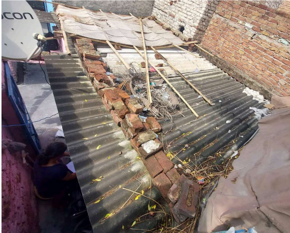
Fig 25.2.1.6-2 : Roof- Top View
