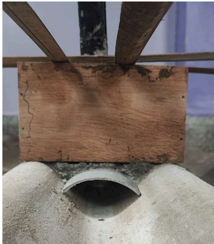
Fig 37.7.2-8 : Casting the support with drip line
