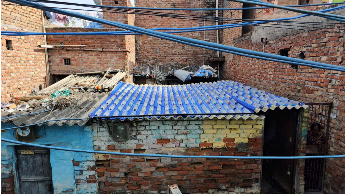
Fig 37.5.3-8 : Final View After MS Strip Installation
