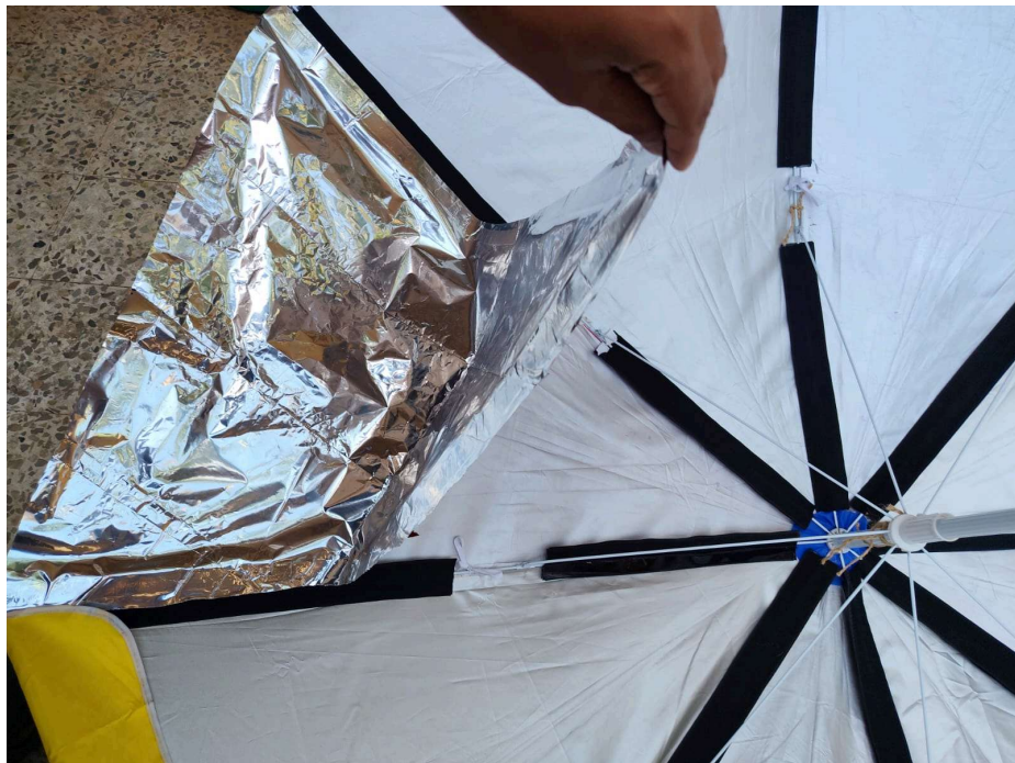
Fig 35.8.1-11 : MLP sheets Bonded Together
