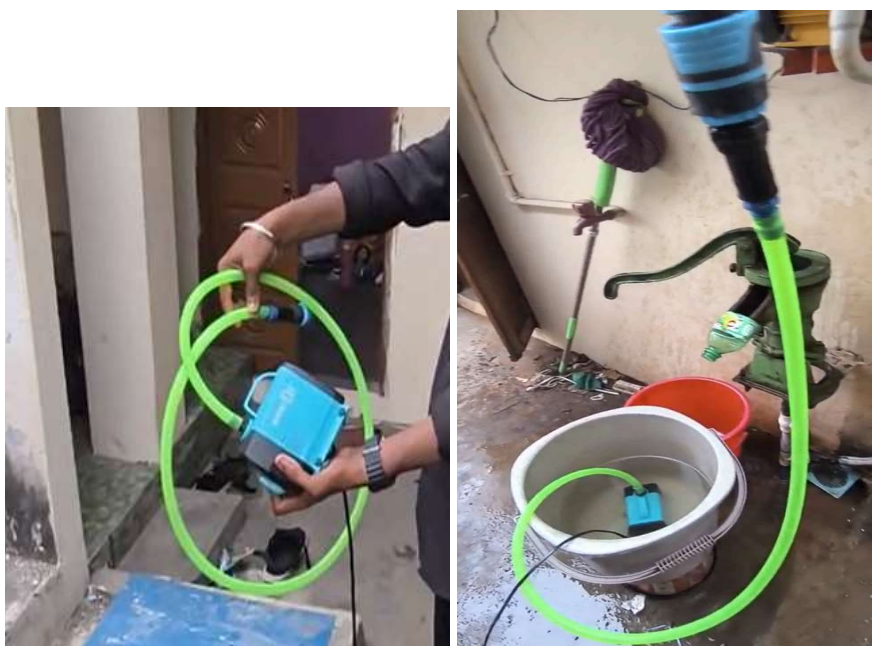
Fig 35.3.2-4 : Submersible Pump Connected with Hosepipe
