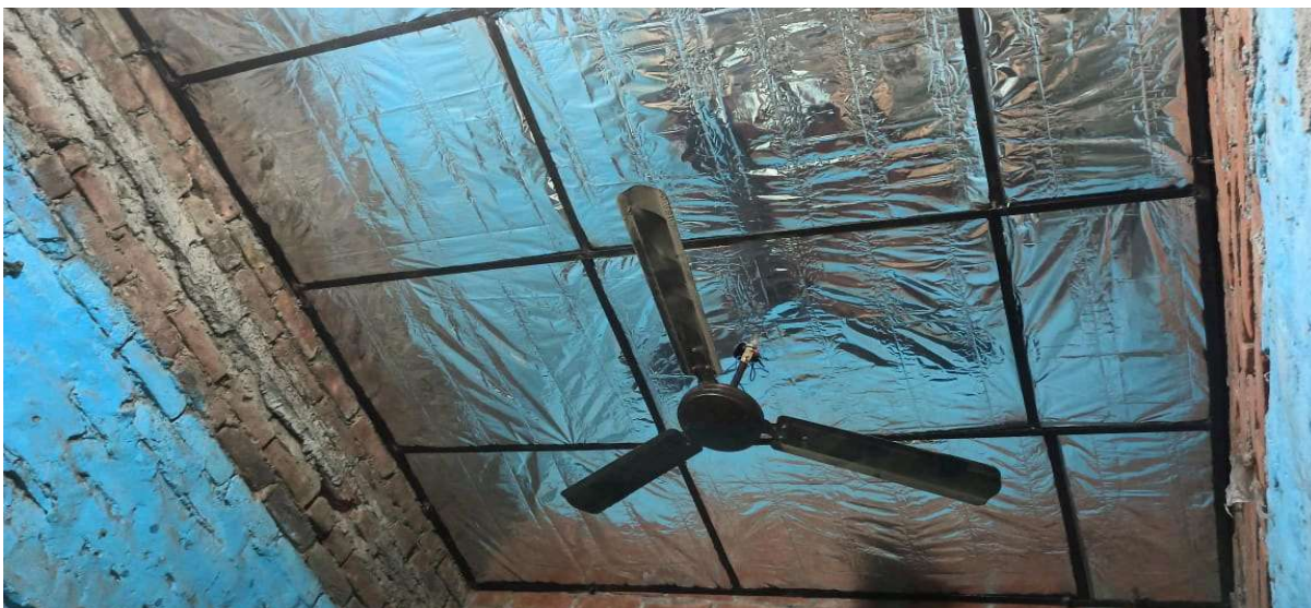
Fig 37.2.5-7 : Metal support framework with panels in place with no gap in the ends
