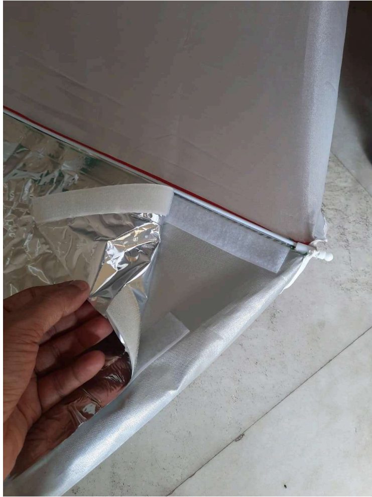
Fig 35.8.1-7 : Attaching of Velcro Strips
