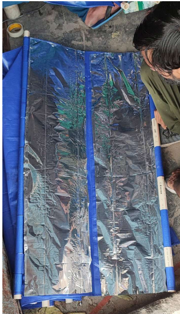
Fig 37.7.2-11 : Attaching MLP to Tarpaulin
