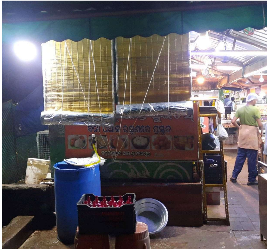
Fig 22.1.2.7-1 : Vertical Cane Blind Installation
