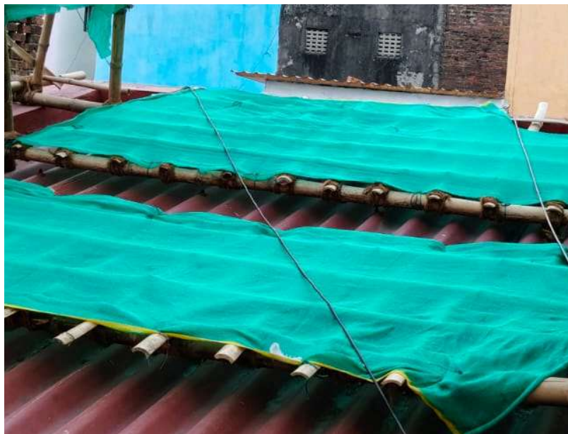
Fig 37.4.2-13 : Trellis after finishing all works
