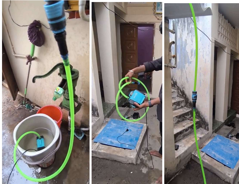
Fig 37.4.2-16 : Submersible installation along with hose pipe
