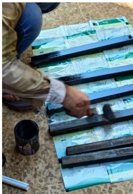
Fig 37.7.2-4 : Painting of Box Sections
