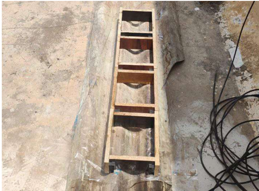
Fig 37.7.2-5 : Placing of moulds on roofing sheet
