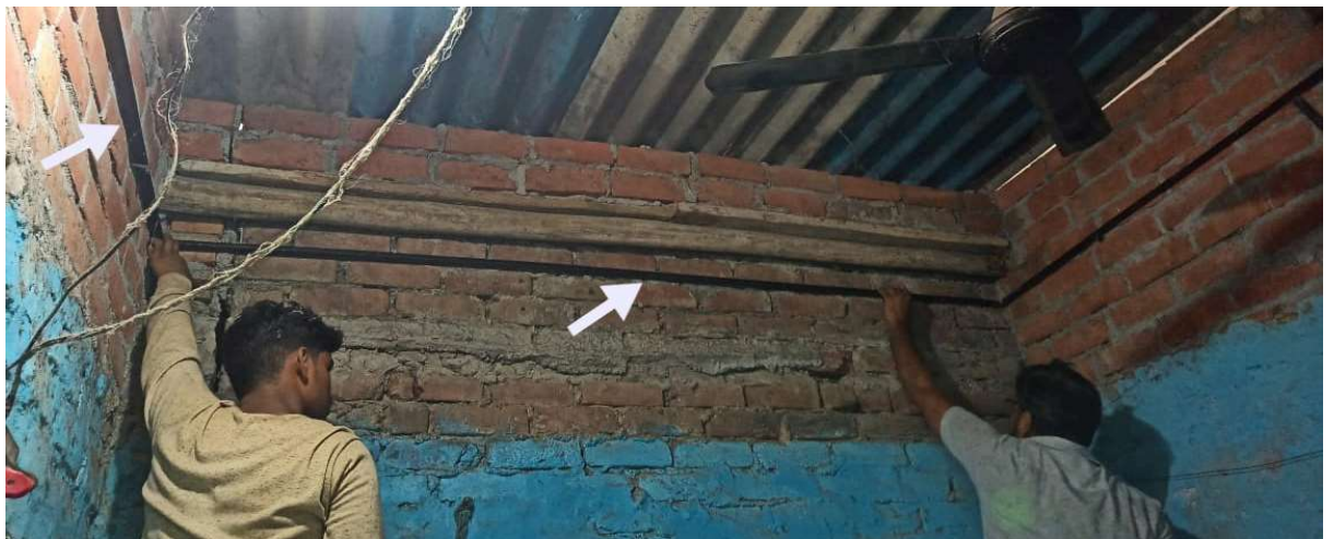
Fig 37.2.5-2 : MS L-angle drilled at a height of 14" approx(in this instance) from top of wall on all 4 walls to form the support frame
