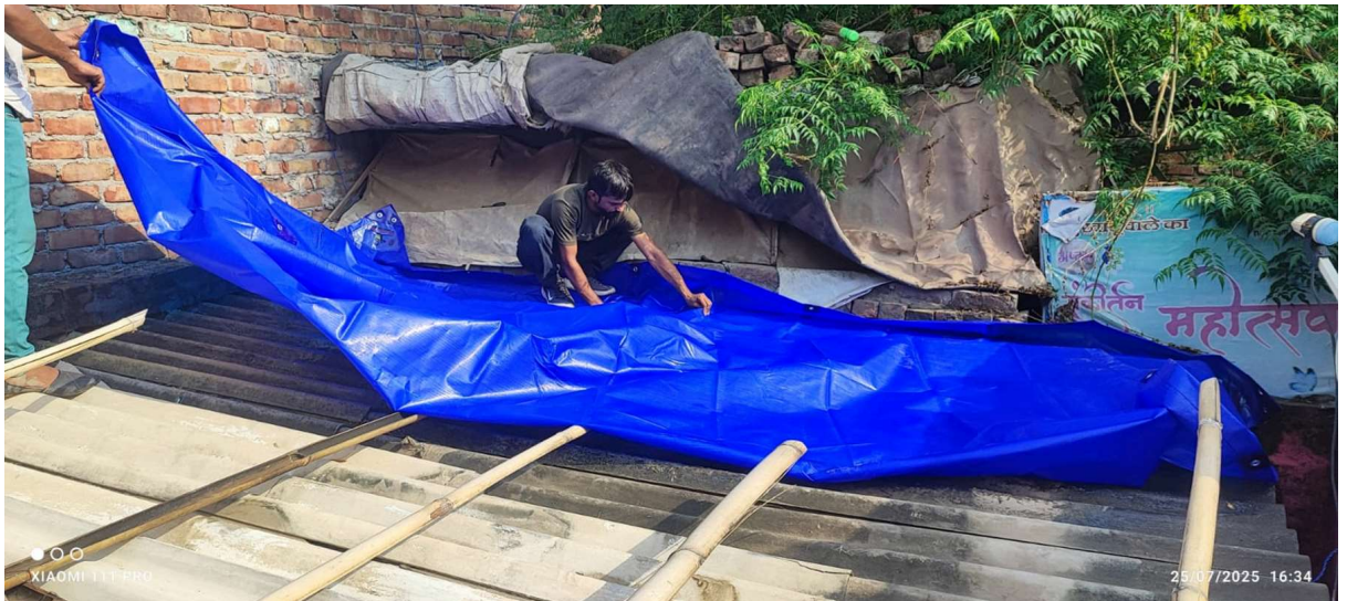
Fig 37.6.3-2 : Placing Of Silpaulin Above Roof
