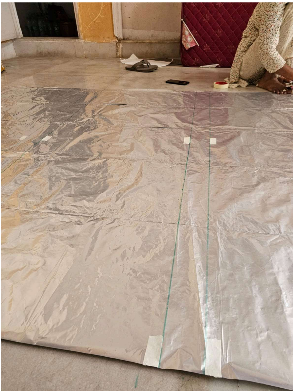
Fig 37.1.2-11 : Placing paper tape for marking 3 inch loop
