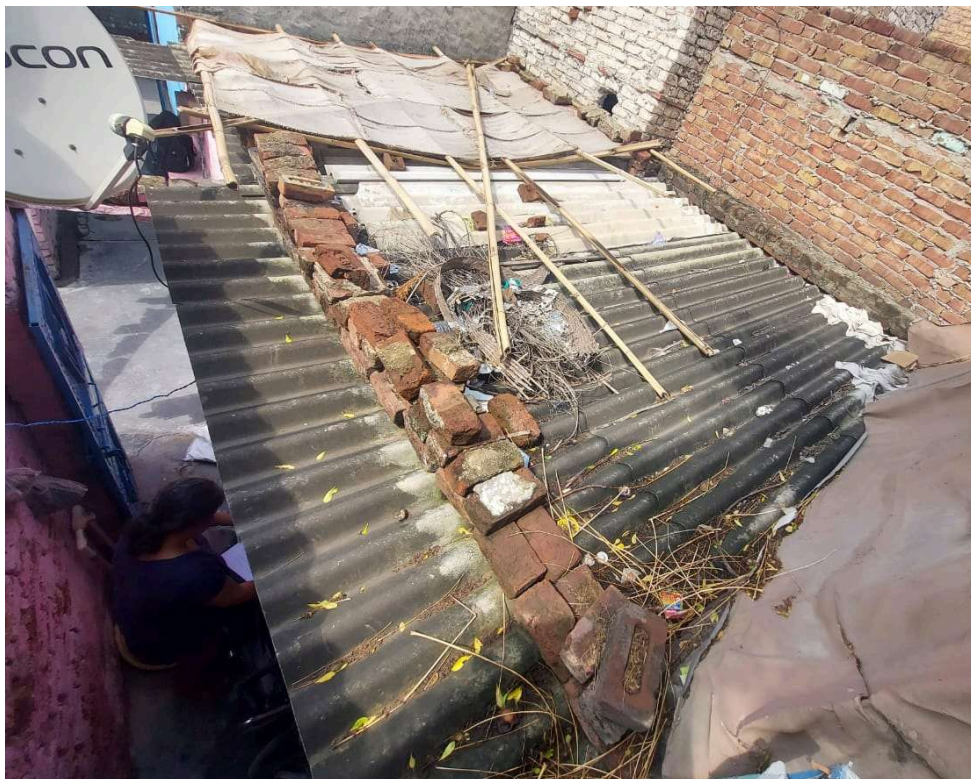
Fig 25.2.1.6-2 : Roof- Top View
