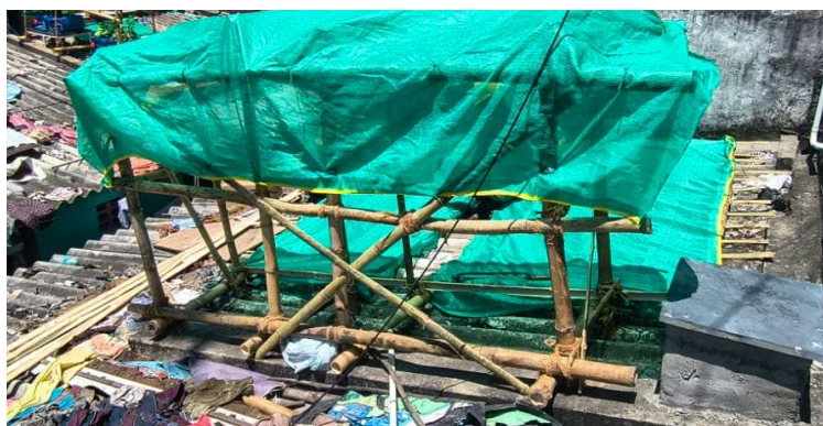
Fig 35.3.3-2 : Scaffolding Structure with Shade Net
