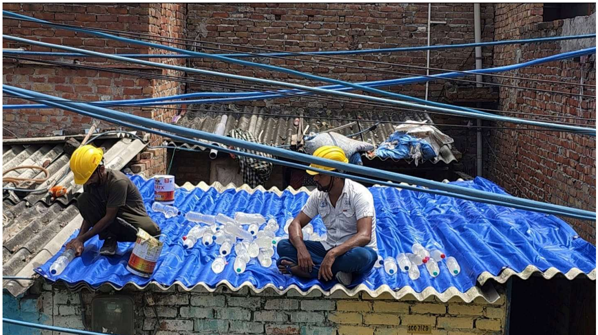
Fig 37.5.3-5 : Placing Of Bottles In The Trough Of Roof With Equal Spacing
