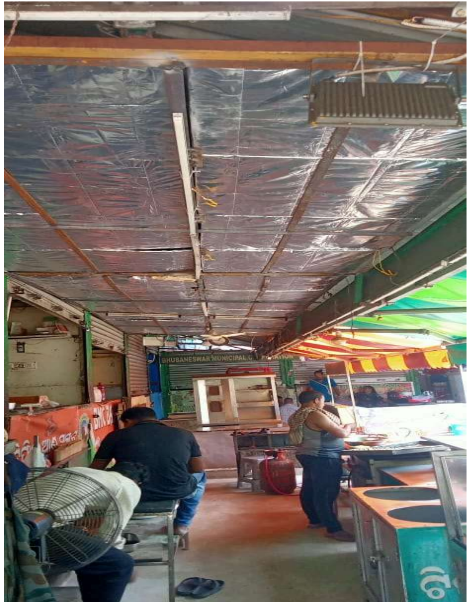
Fig 22.1.2.7-2 : Biomass Panel Installation
