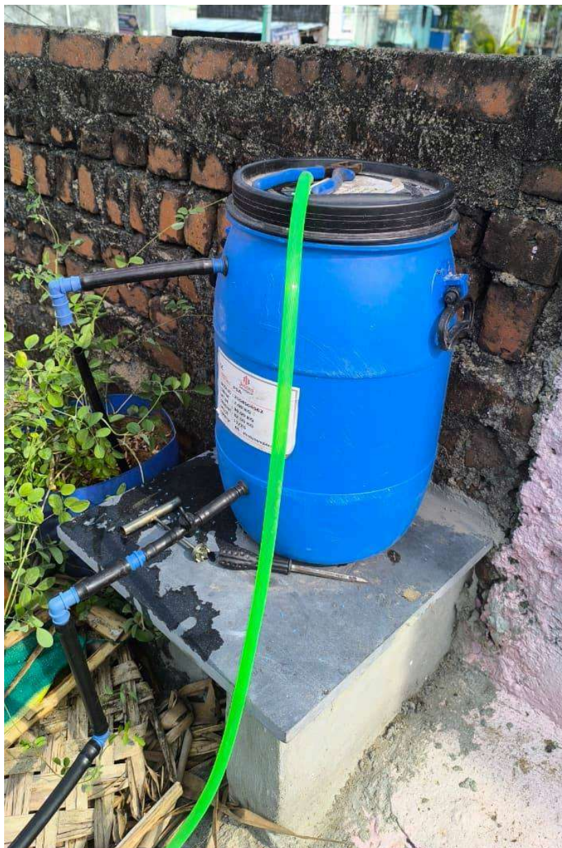
Fig 37.4.1-1.5-1 : Over Head Tank After Installation
