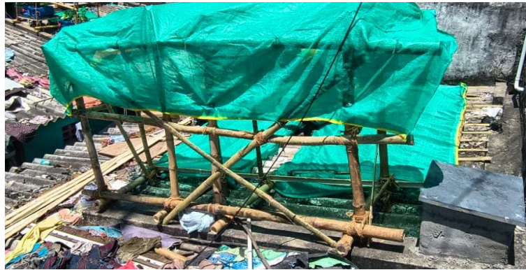
Fig 37.4.2-15 : Scaffolding after finishing all works
