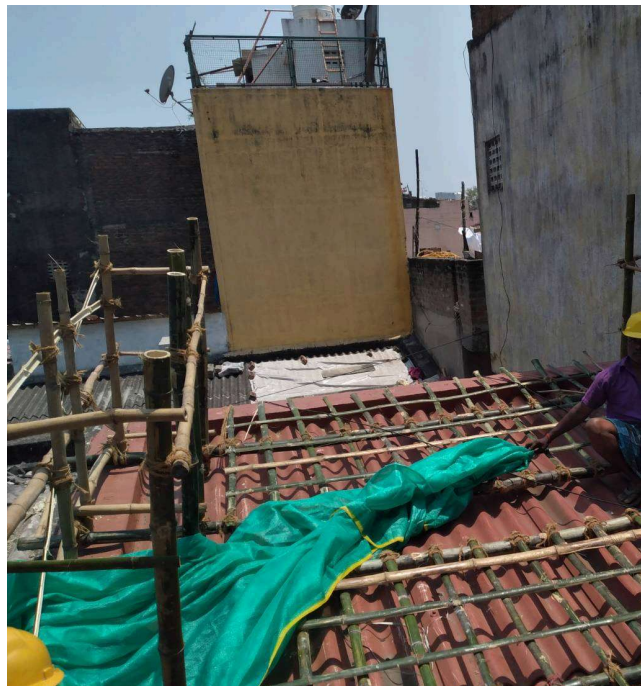
Fig 37.4.2-12 : Green net attaching to the Bamboo trellis
