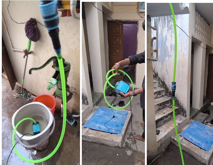
Fig 37.4.2-16 : Submersible installation along with hose pipe
