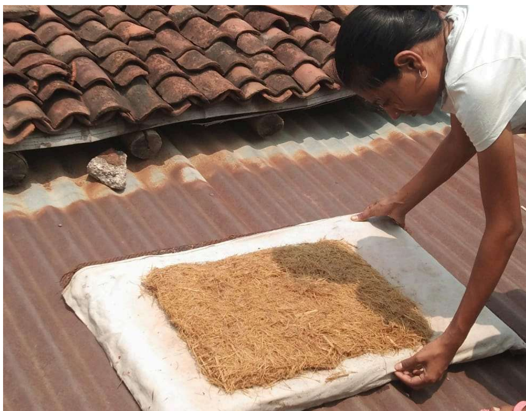
Fig 37.2.2-12: Sun-dry the panels
