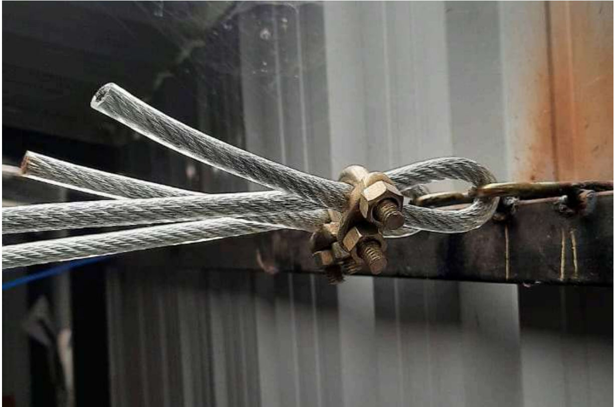
Fig 37.1.2-4 : Establishing wire rope to wall using U-clamps
