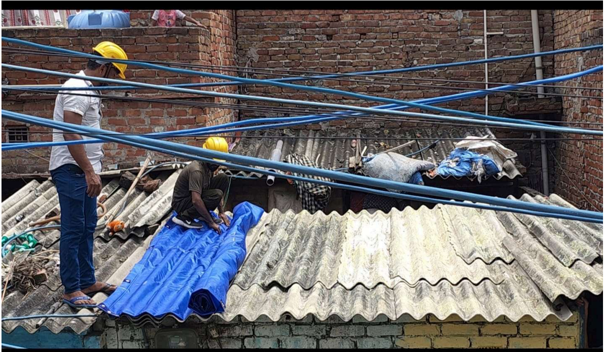
Fig 37.5.3-2 : Sticking Of Silpaulin Across The Roof
