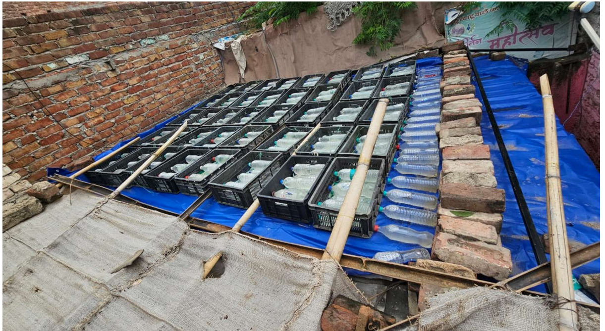
Fig 37.6.3-6 : Final Placement Of Pet Bottle In Crates
