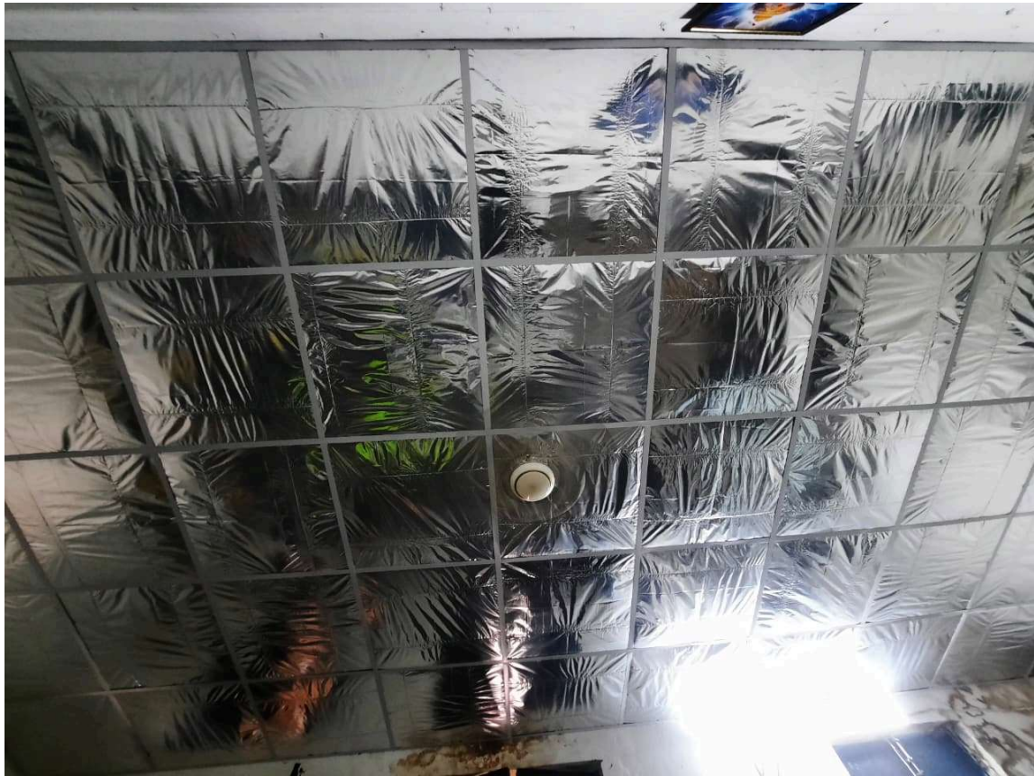
Fig 22.1.6-1 : MLP Static Panel Installation at Office Space
