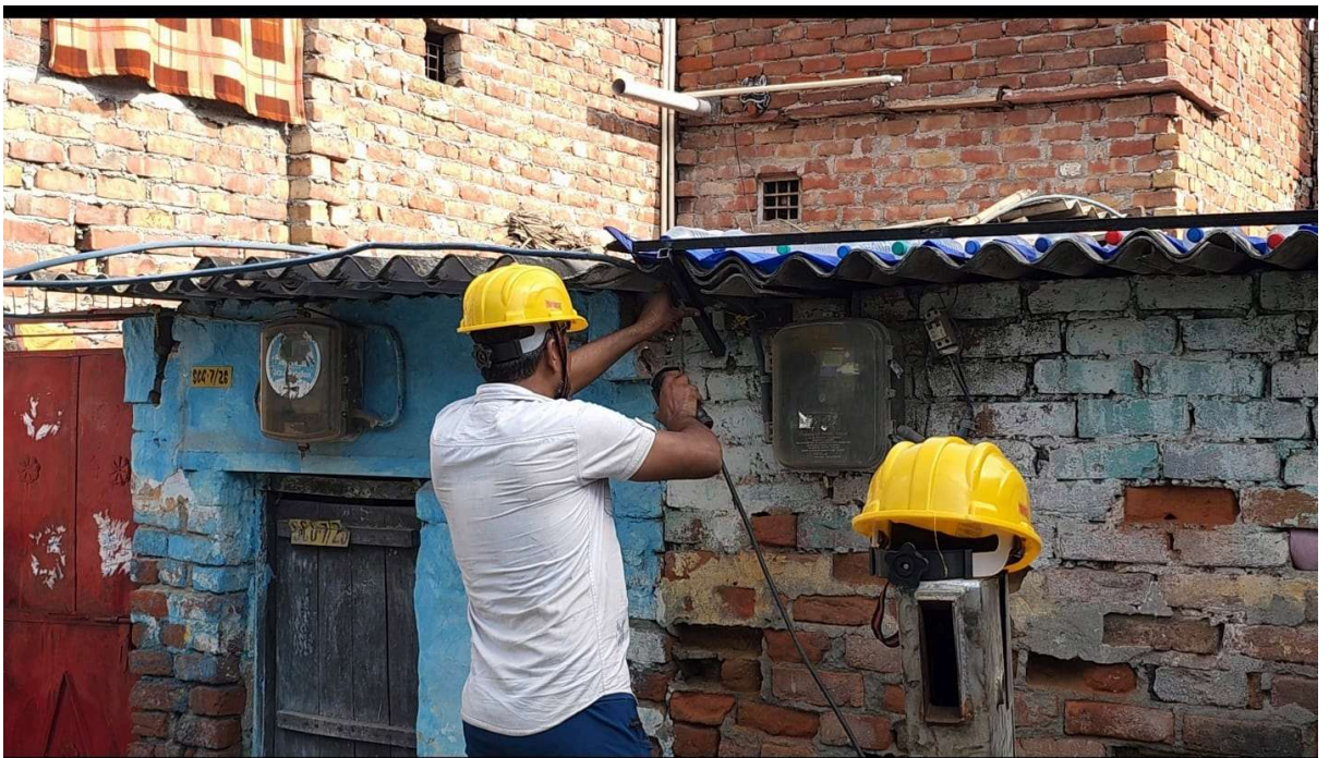
Fig 37.5.3-7 : Securing Of MS Strip Through Welding
