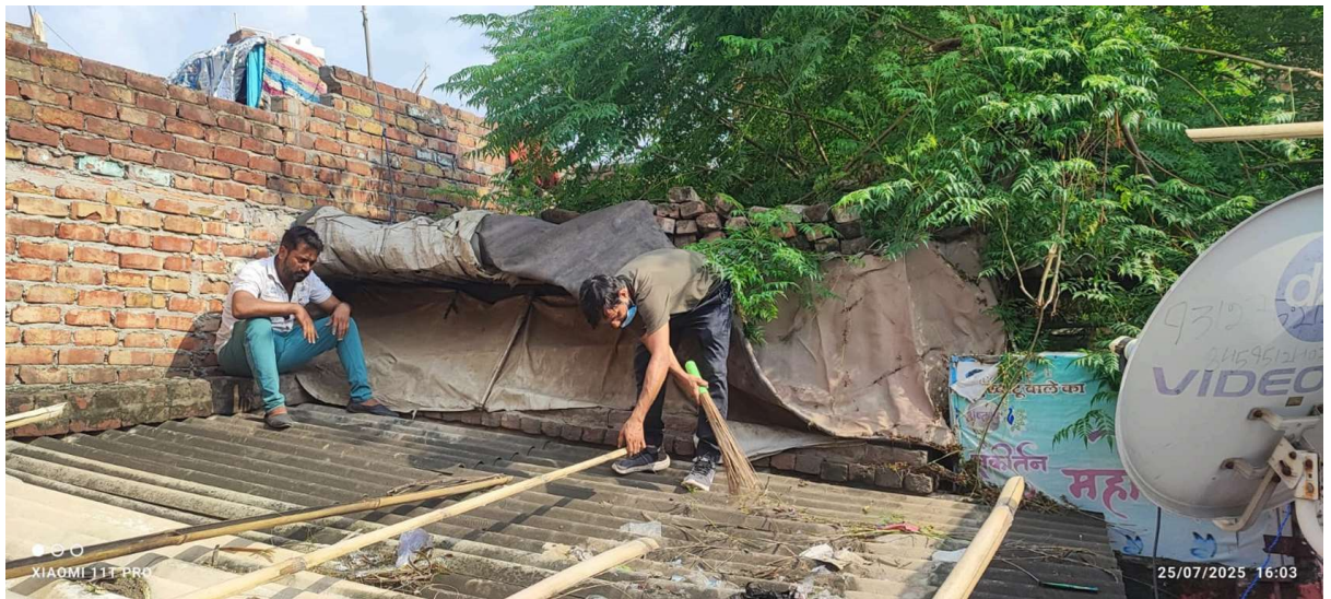
Fig 37.6.1-1 : Cleaning Of Roof
