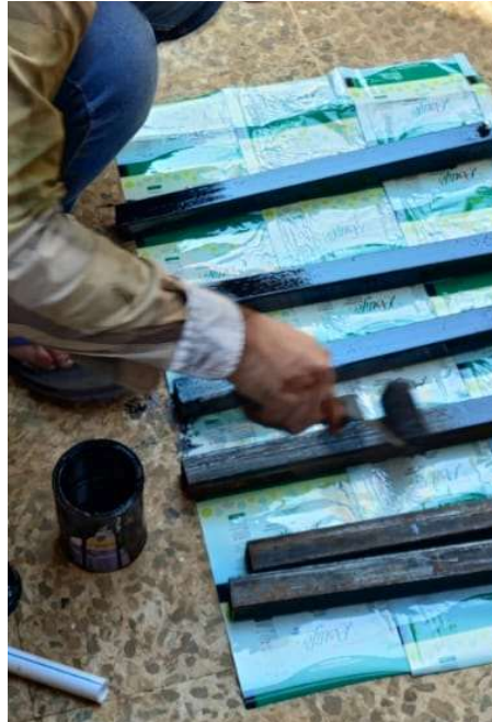
Fig 37.7.2-4 : Painting of Box Sections
