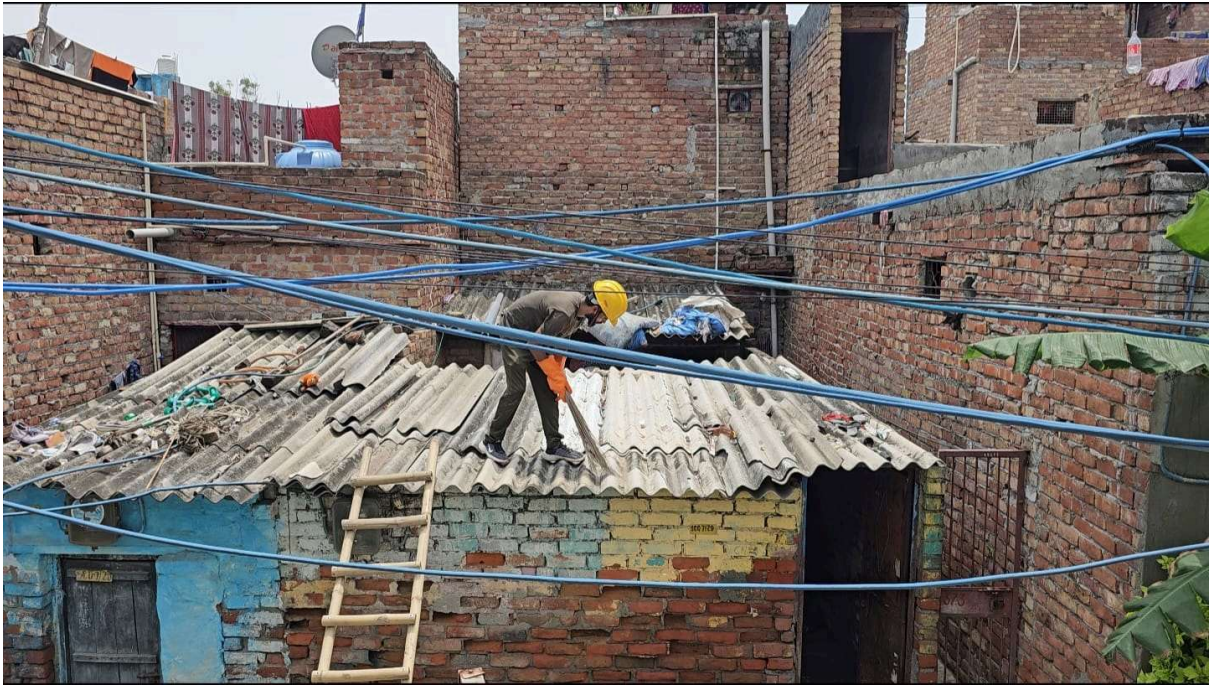
Fig 37.5.1-1 : Cleaning Of Roof
