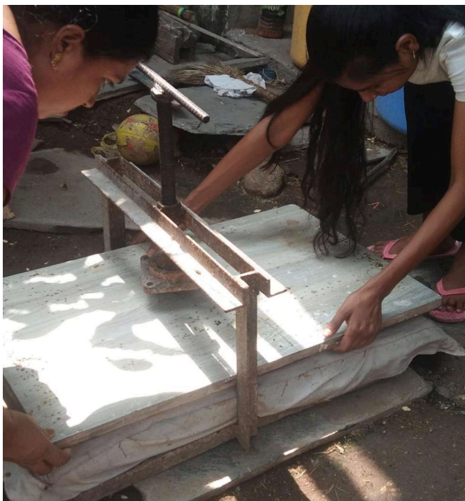
Fig 37.2.2-11: Press the panels to remove excess water
