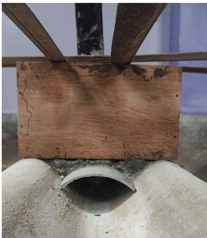
Fig 37.7.2-8 : Casting the support with drip line
