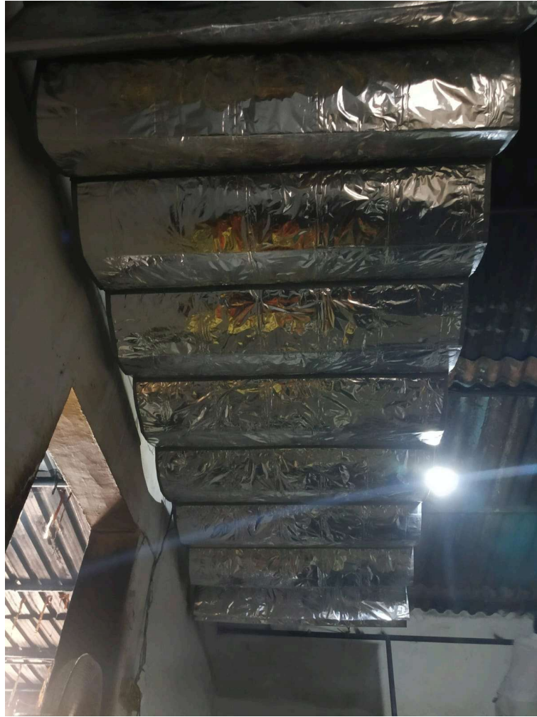
Fig 22.1.1.11-1 : Internal Radiant Barrier Installation
