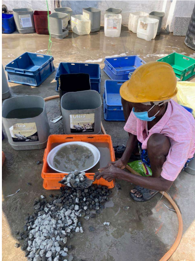
Fig 37.4.2-6 : Washing concrete chips
