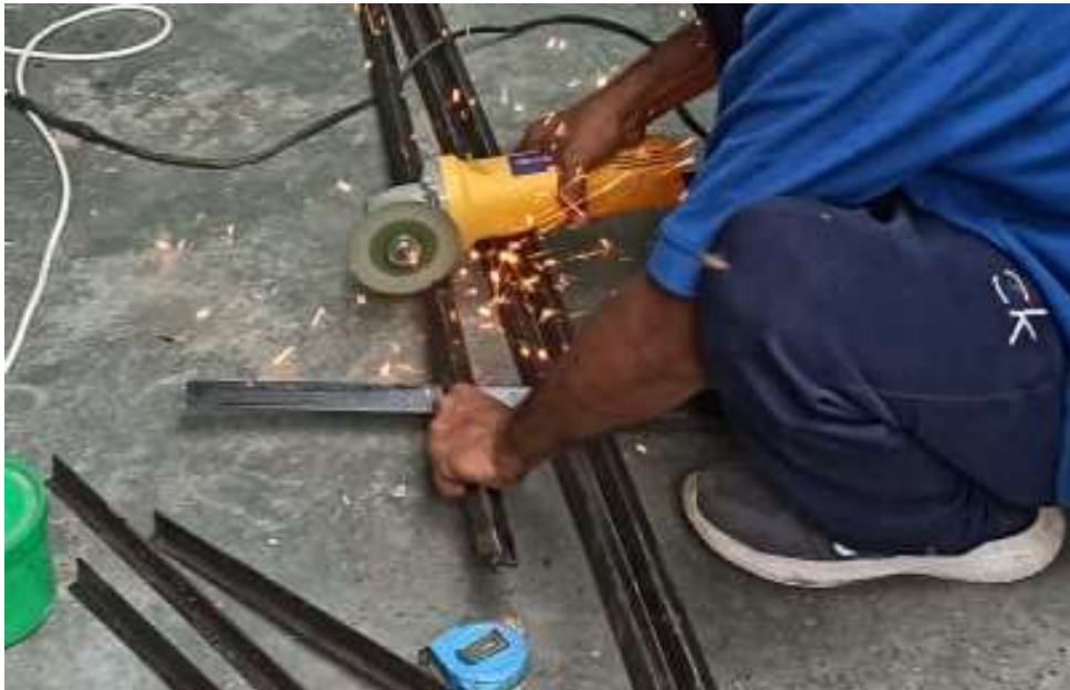
Fig 37.2.5-1 : MS L-angle lengths being prepared for panel support frame
