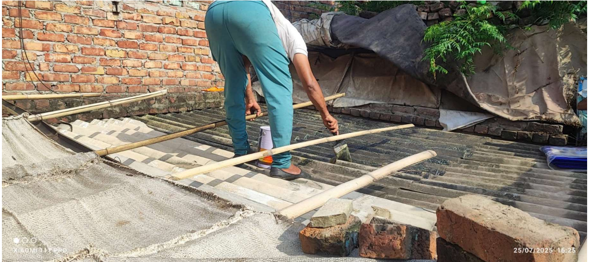
Fig 37.6.3-1 : Applying Of Adhesive Above The Roof
