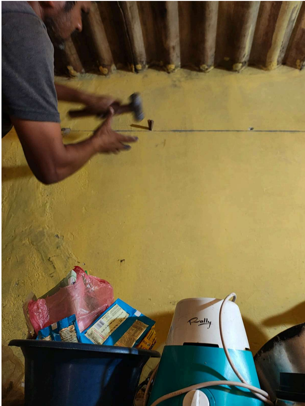
Fig 37.8.3-1 : Marking on the wall
