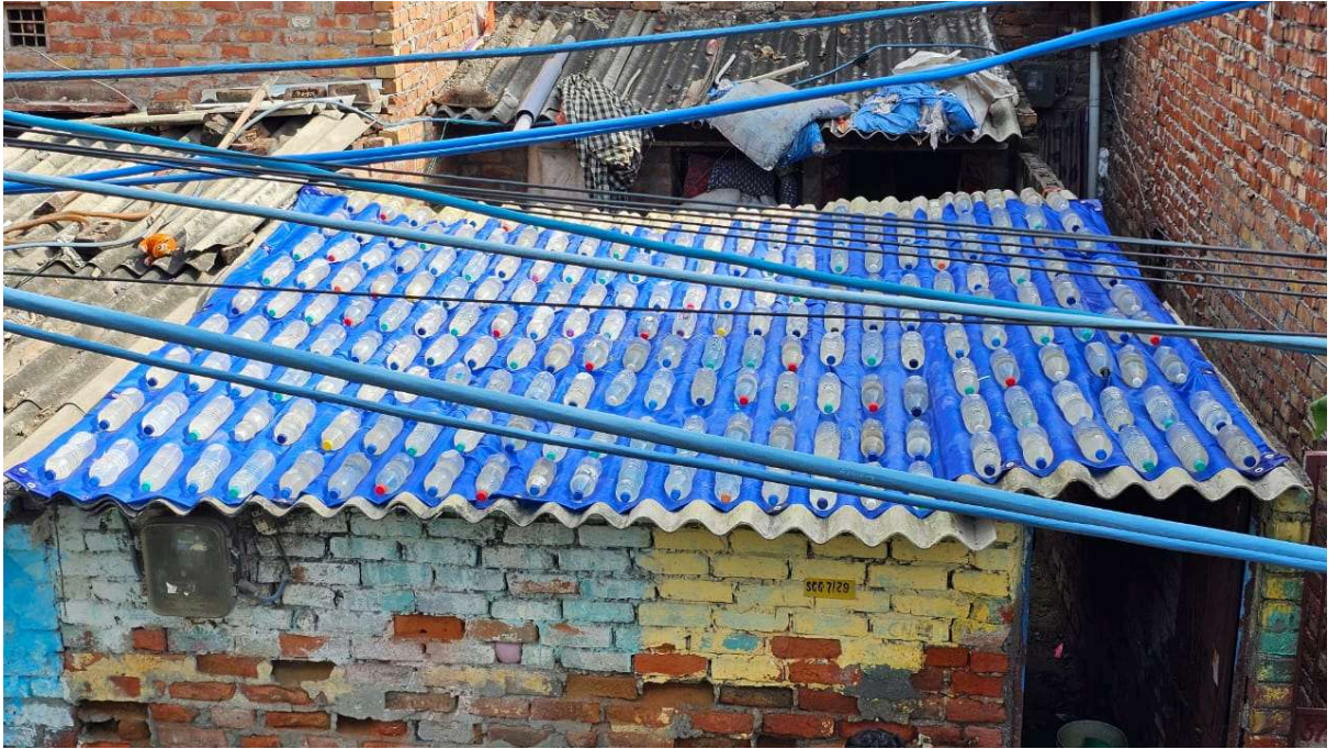
Fig 37.5.3-6 : Final View After Placing Of PET Bottles
