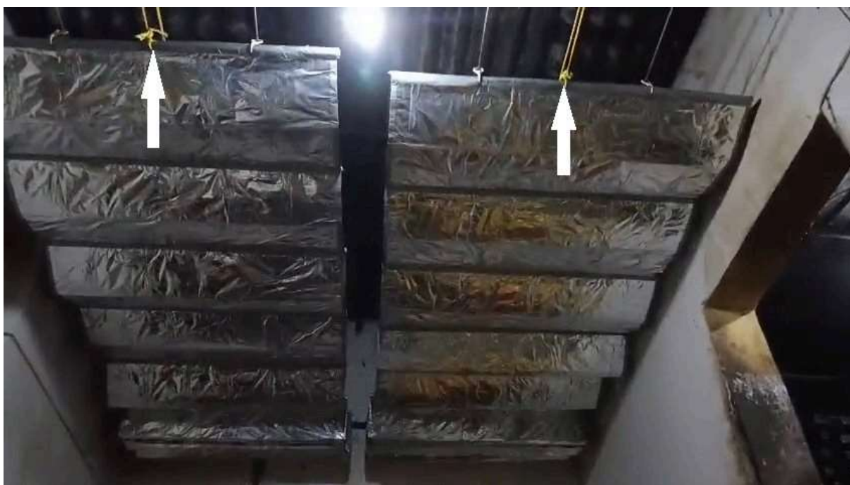
Fig 37.1.3-5: Attaching nylon rope to the front end pipe of the fractal
