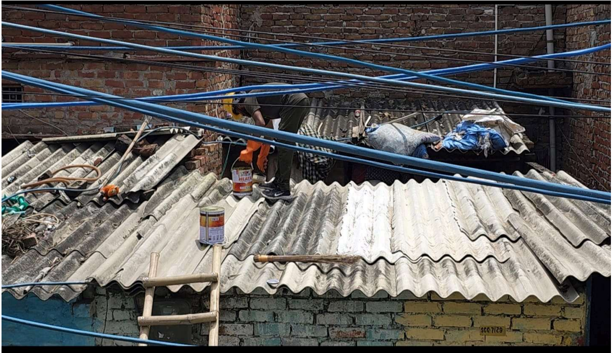
Fig 37.5.3-1 : Applying Of Adhesive Over The Roof
