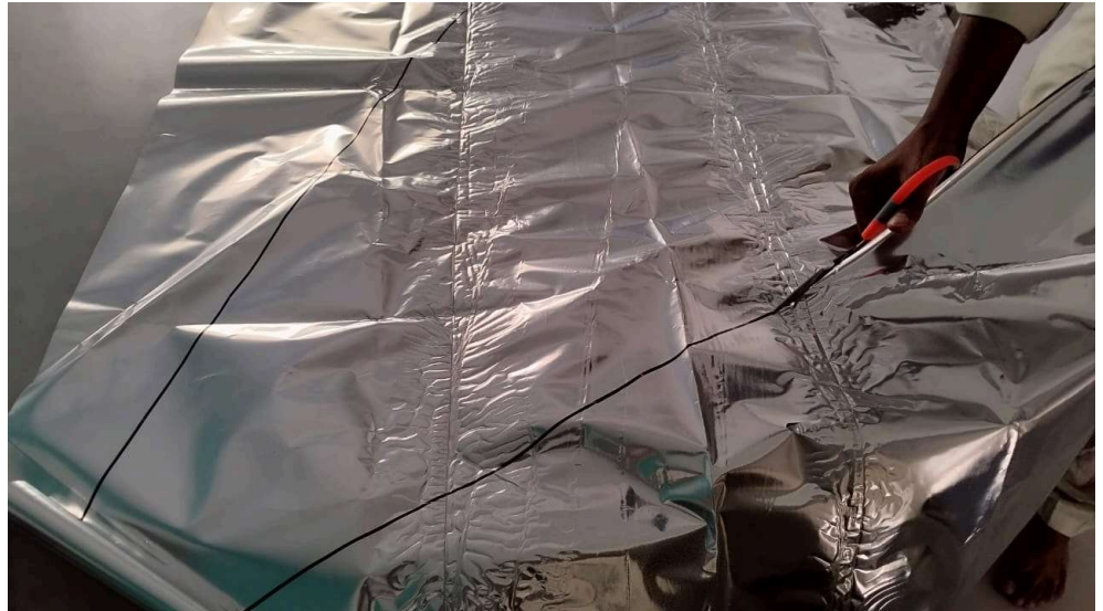
Fig 37.9.2.1.4-1 : Cutting of Mlp according to measurements taken
