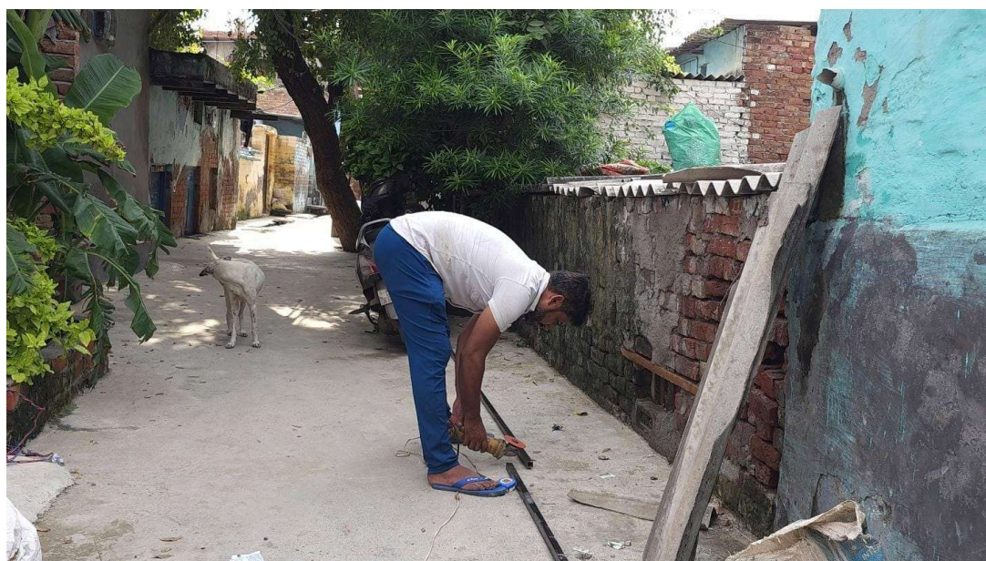
Fig 37.5.2-2 : Cutting Of MS Strip
