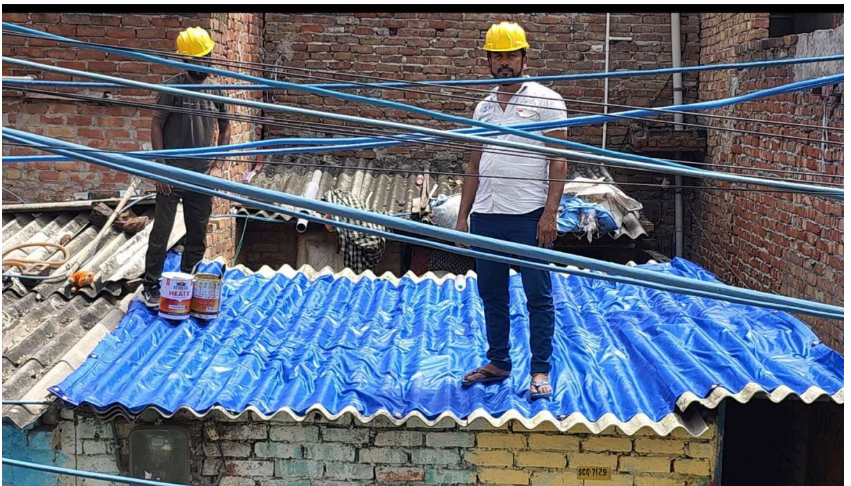
Fig 37.5.3-3 : Final View After Application Of Silpaulin
