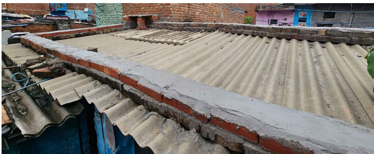
Fig 37.4.1-1 : Parapet wall after repair works
