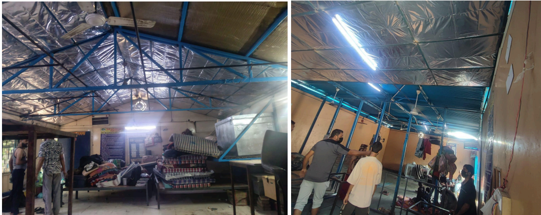
Fig 8: Panels Installation
