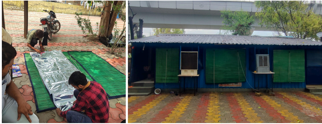
Fig 9: Vertical Cane Blinds Installation
